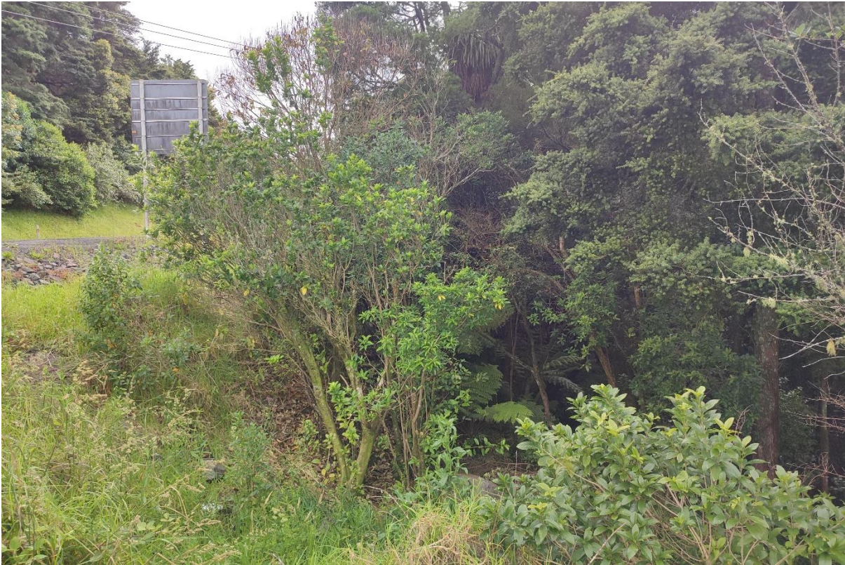
Figure 13. Bank from roadside drops very steeply to the right in this image, dam (R09/2263) is located below in the bush.
