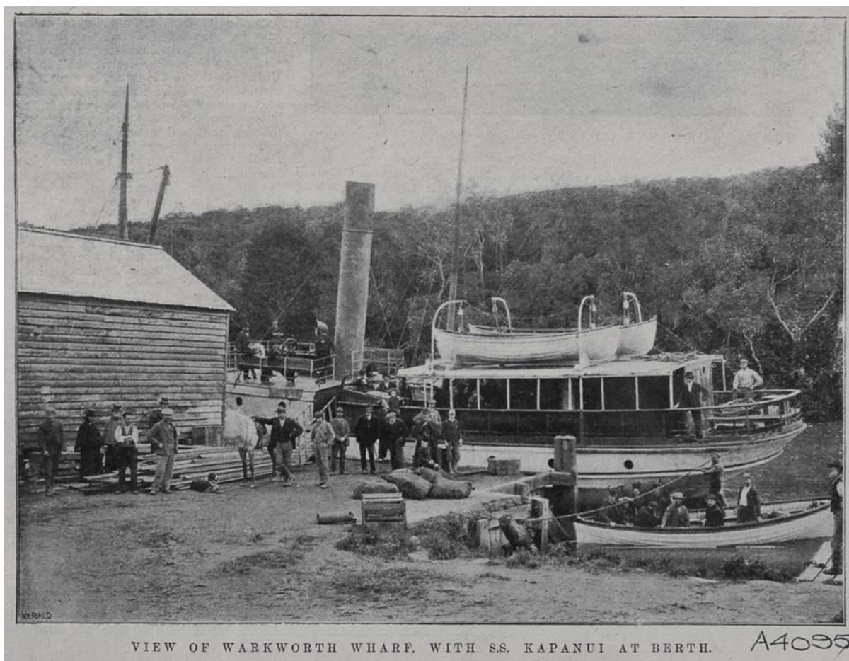
Figure 3. View of the Warkworth Wharf from Auckland Weekly News, c. 1890 – 1899. https://digitalnz.org/records/30086952/view-of-the-warkworth-wharf-with-ss-kapanui-at-berth
