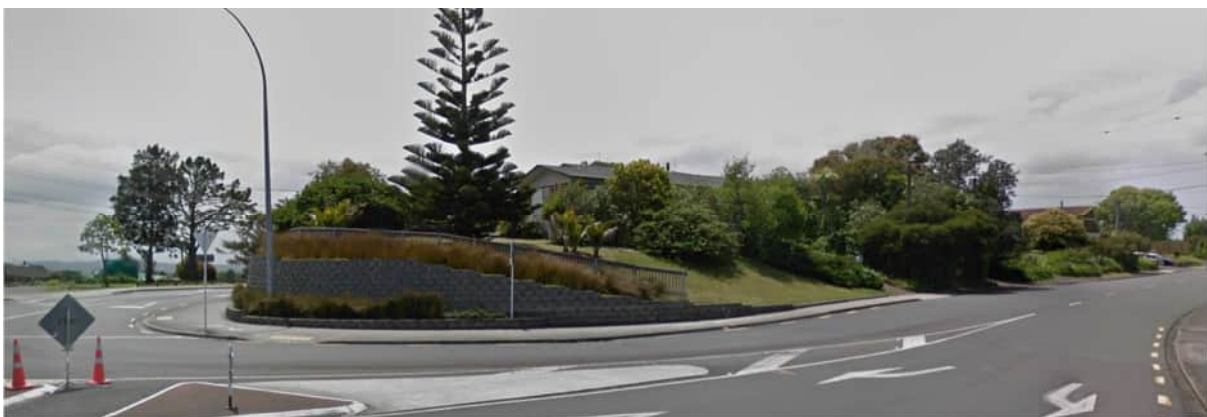
Figure 7: Existing retaining wall feature and buffer planting at Don Buck Road / Royal Road intersection
