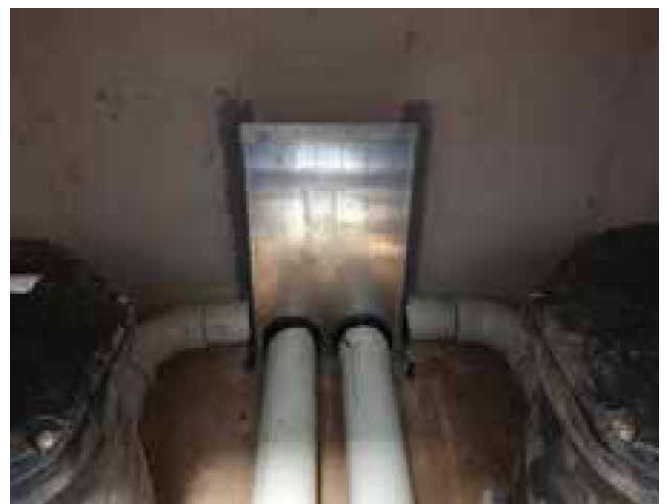
Figure 3 - Typical Outlet Weir Wall
