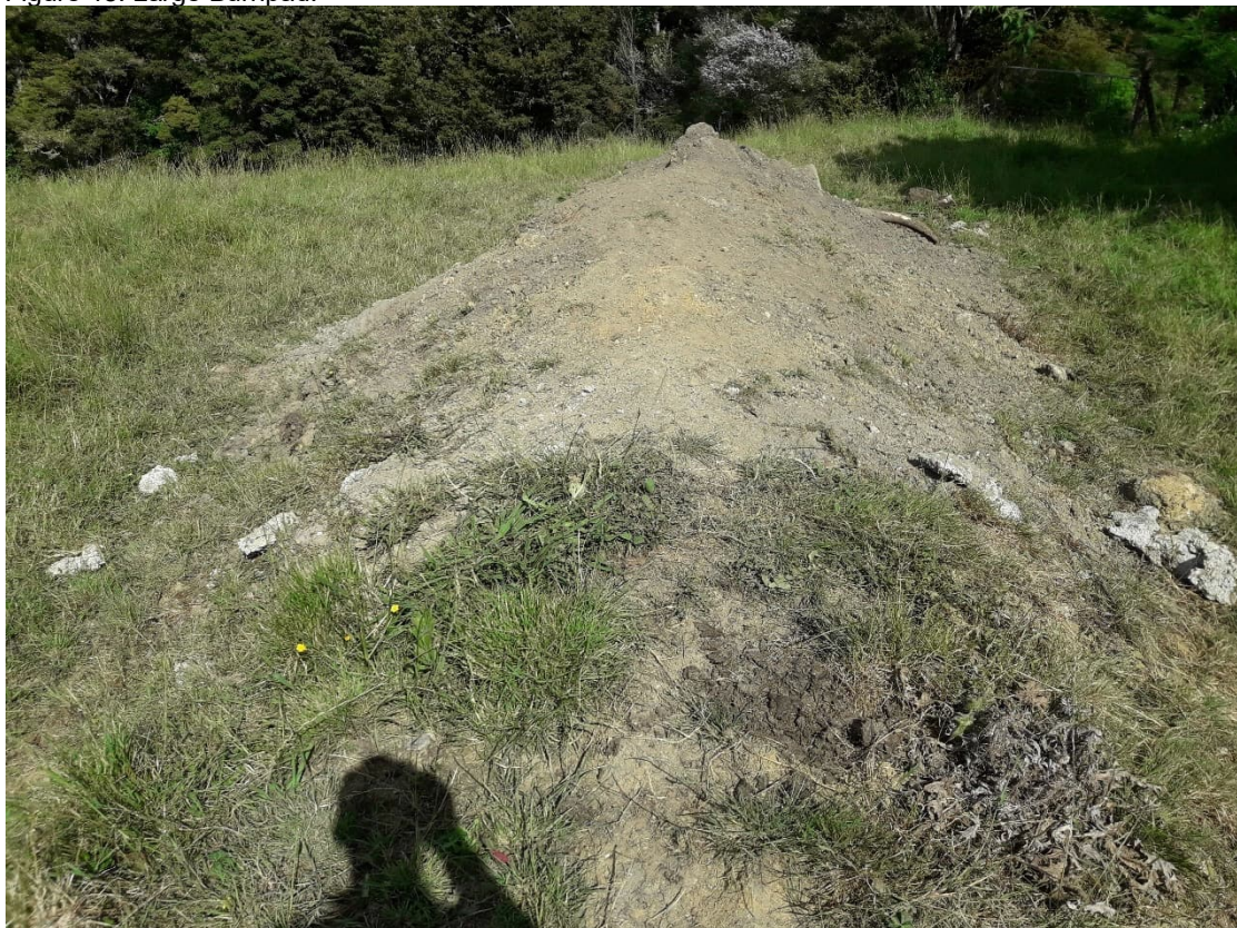
Figure 19: Soil stockpile including concrete rubble.
