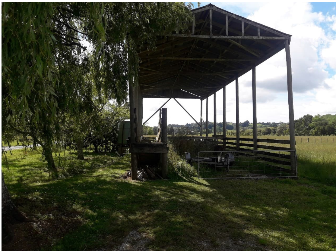
Figure 25: Covered stock yards. Treated timber construction.
