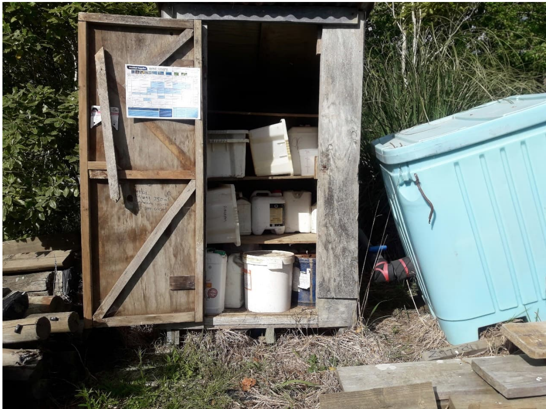
Figure 16: Spray storage shed. Timber construction.
