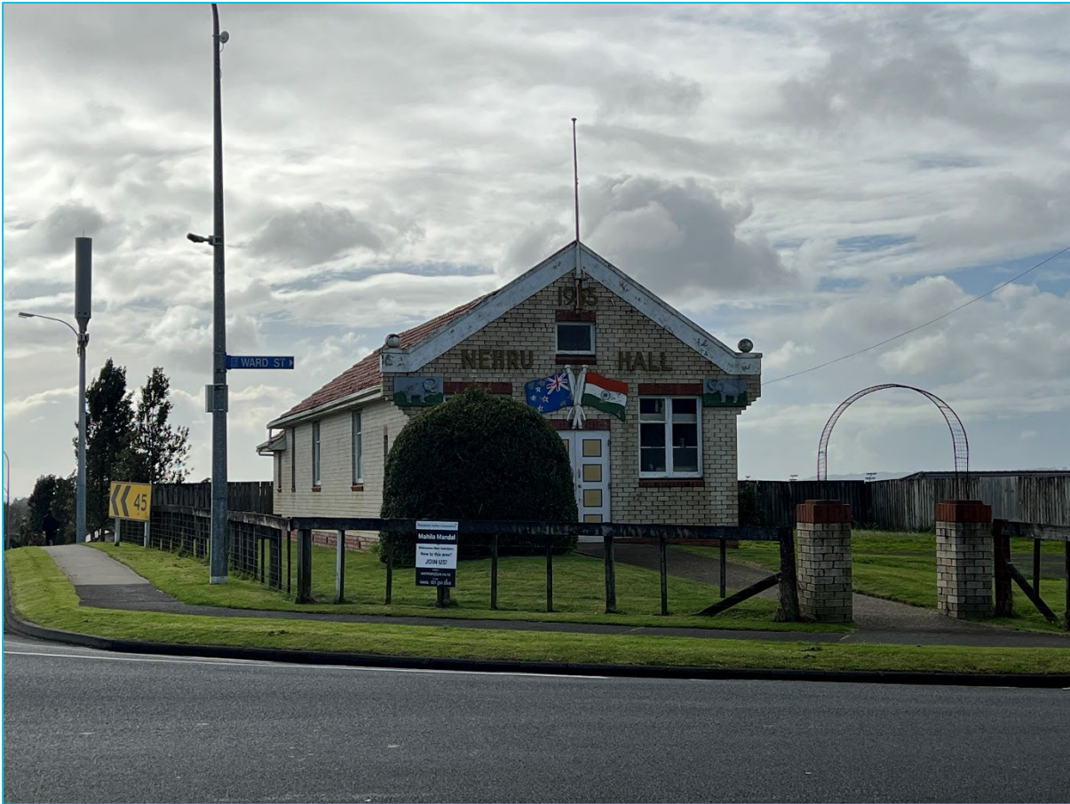
Figure 4-3: Nehru Hall, showing the brick gateway that sits inside the NoR 6 designation.
