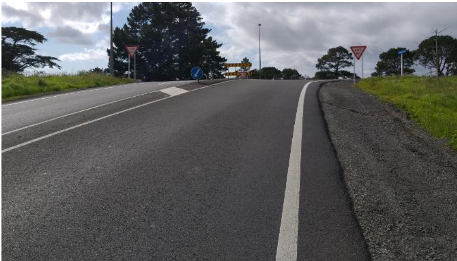
Source: MM site photograph – Pine Valley Road southbound towards the Dairy Flat Highway intersection
