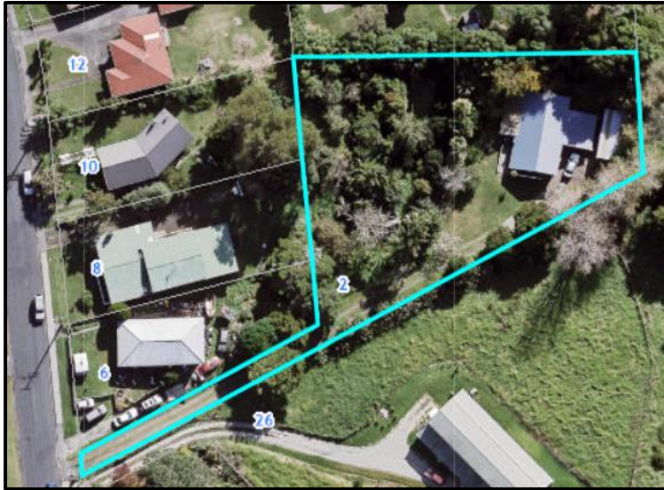
Figure 13: Aerial image of 2 Monowai Street, Wellsford Image courtesy of Auckland Council GIS Maps
