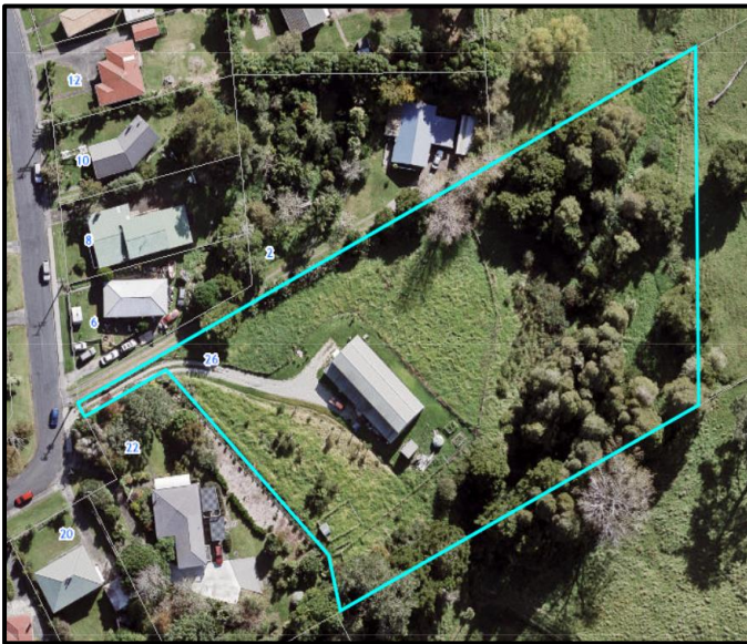
Figure 12: Aerial image of 26 Batten Street, Wellsford
