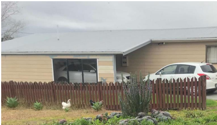
Image 2: Second dwelling 11 Wi Apo Place visible to east of fibrolite dwelling, of hardiplank construction with iron roof.
