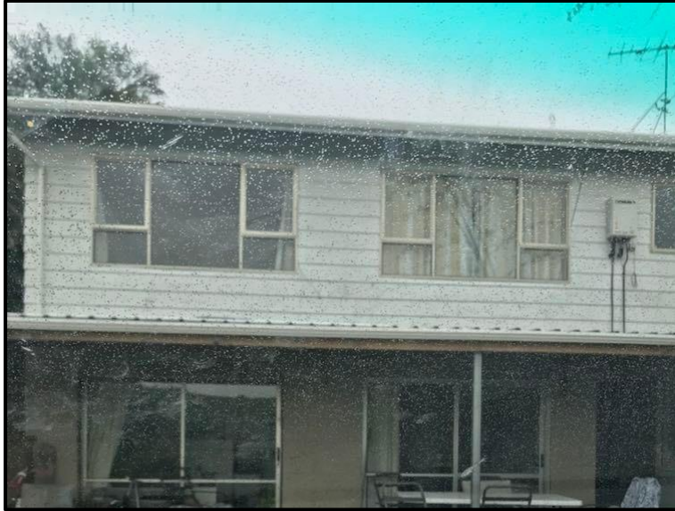
Image 7: Dwelling at 18 Monowai Street, Wellsford
