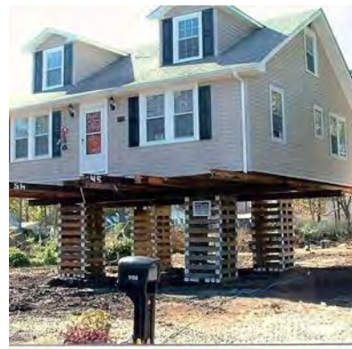
House on temporary bearers
