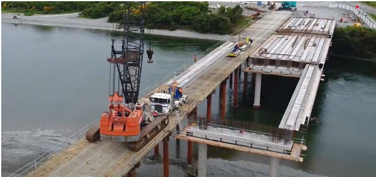
Figure 4 - Typical temporary staging – the orange crane and truck are sitting on the temporary staging. The new bridge is to the right
