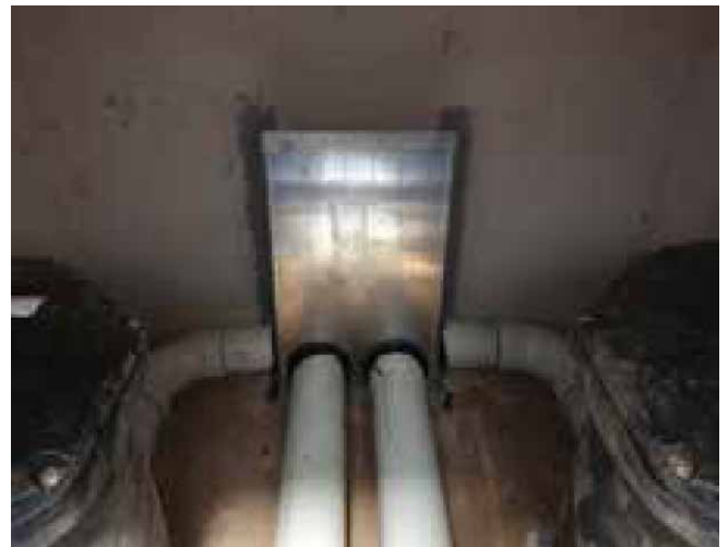
Figure 3 - Typical Outlet Weir Wall
