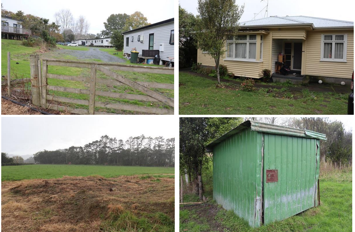
Figure 60. Top left: Modern dwellings (units) on south side of property P5, facing south. Note, the ones on the left and right are contained within P5 while the ones in the background are contained within P6. Top right: older (c. mid-20th century) house on the south side of property P5, facing west. Bottom left, fields on the north side of P5 showing flat terrain, facing northwest. Bottom right: Old corrugated iron shed on the east side of P5, facing south
