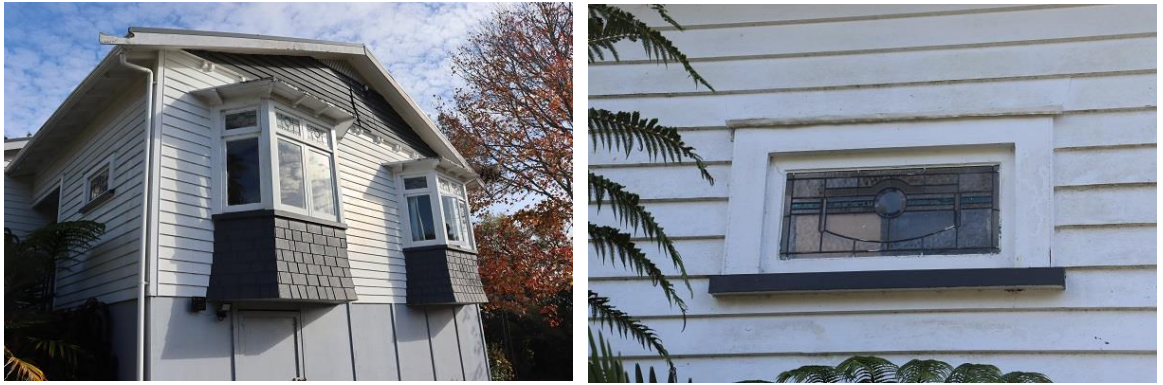
Figure 94. Left: Oriel style windows of c.1920s/1930s house located on the northwest side of P7, facing northwest. Right: Close-up view of one of the small decorative windows, facing north. This example is located on the south wall of the building, east side
