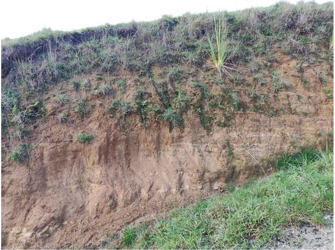
Figure 121. Profile of hill from track cut into hill. Note the stratigraphy here. Facing east
