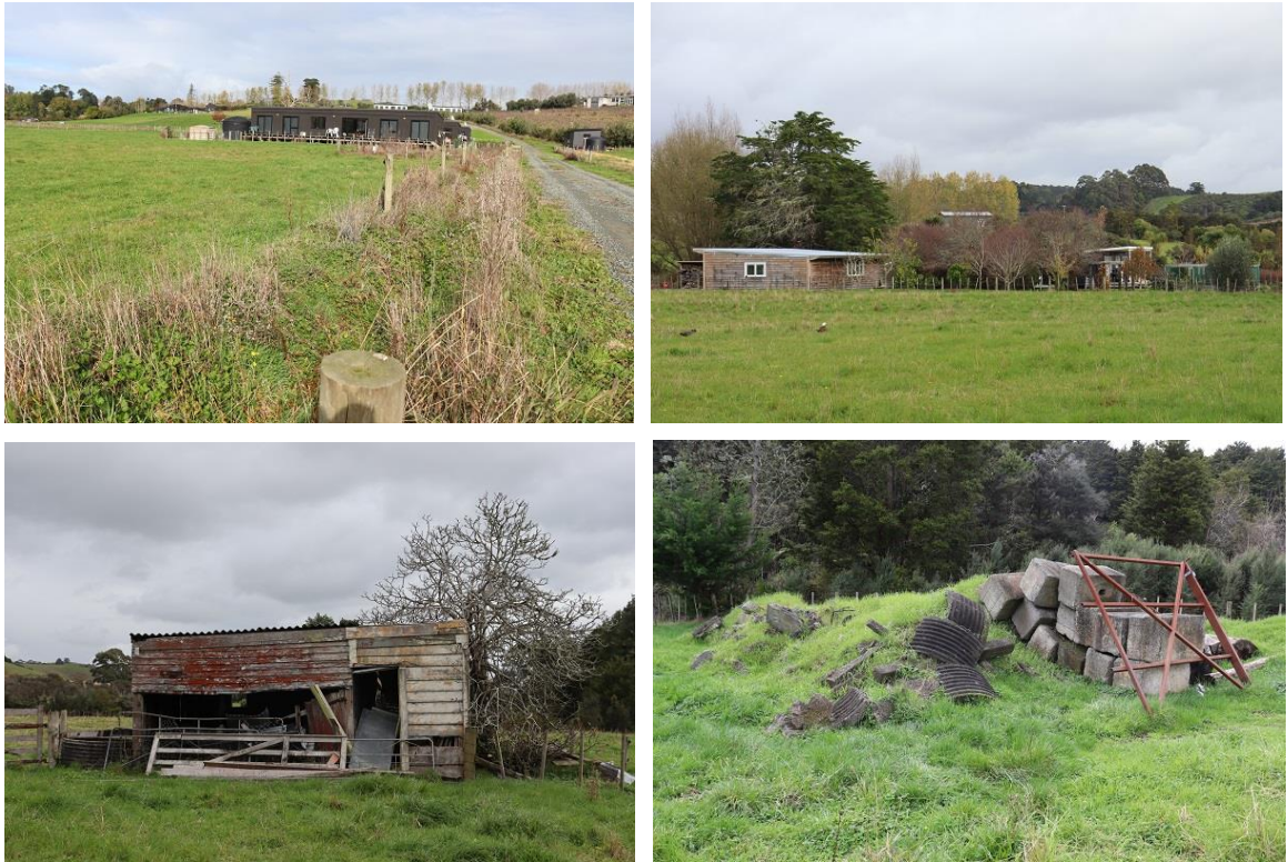
Figure 57. Top left: Modern dwellings (units) located on the southern side of P4, facing south. Top right: modern dwelling at the centre of property P4 with adjacent barn/shed, facing west. Bottom left: Old dilapidated barn on the central northern side of property P4, facing west. Bottom right: Large pile of concrete rubble, blocks and steel framing on central northern side of P4, facing north
