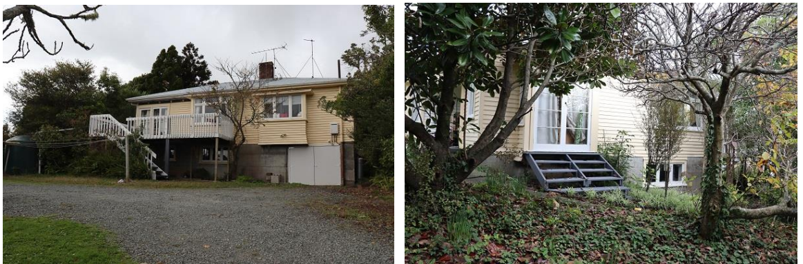
Figure 95. Left: West side of mid-20th century house located on the southeast side of P5, facing south. Right: North side of the same house, facing west.
