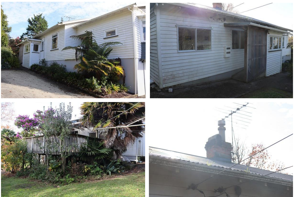
Figure 93. Top left: The c.1920s/1930s house located on the northwest side of P7, facing northwest. Top right: The same house, facing northeast. Bottom left: The same house, facing south. Bottom right: Chimney of the c.1920s/1930s house, facing north/northeast
