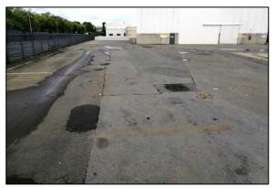
Photo 5: Patched asphalt north of the tank farm building.
