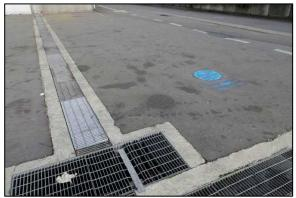
Photo 6: Stormwater drainage system in central area of site between the tank farm building and the 'flexi station.'
