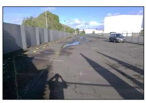
Photo 2: Central eastern area of site showing asphalt car parking area in worn condition.
