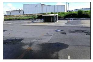
Photo 3: Central yard showing patched asphalt pad.
