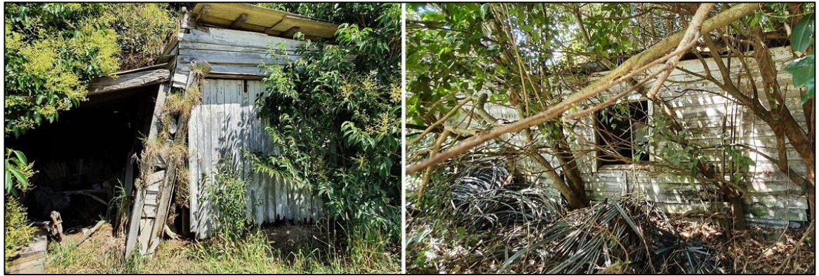
Figure 36. The lean-to structure (left) attached to the small weatherboard hut / cottage structure (right)
