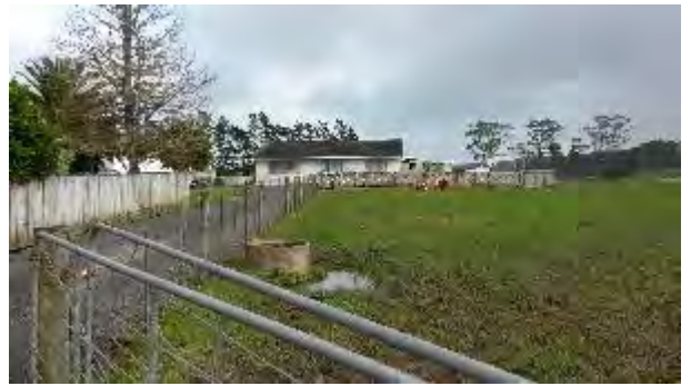
Photo 2: Residential dwelling, facing west.
