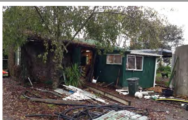
Photo 14: Workshop, facing north west.
