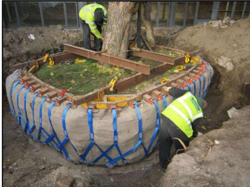
Figure Error! No text of specified style in document.-1 Example showing the lifting, the root ball and the steel frames.
