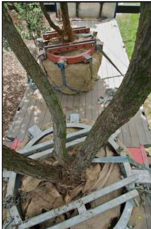
Figure Error! No text of specified style in document.-2 - Example showing the lifting, the root ball and the steel frames.
