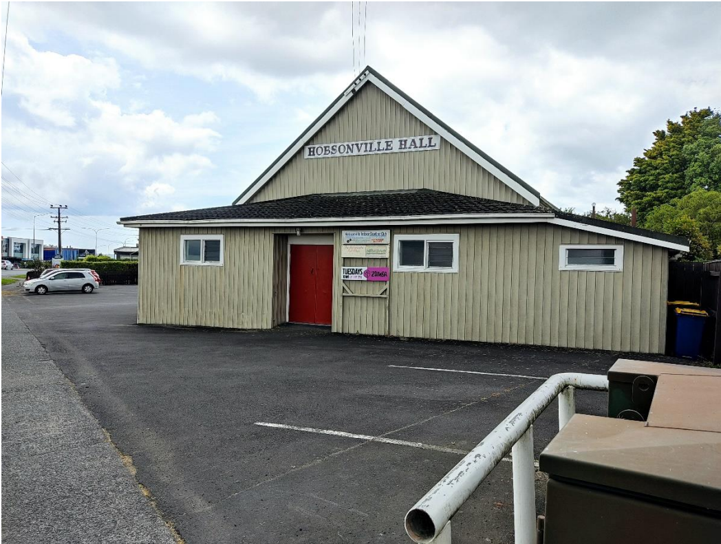
Figure 42: Hobsonville Hall (005) viewed from the road.
