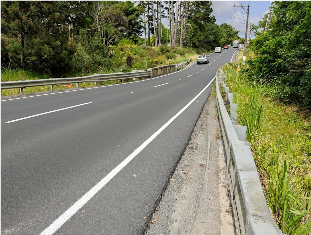
Figure 20: Narrow bridge over the Totara Creek.
