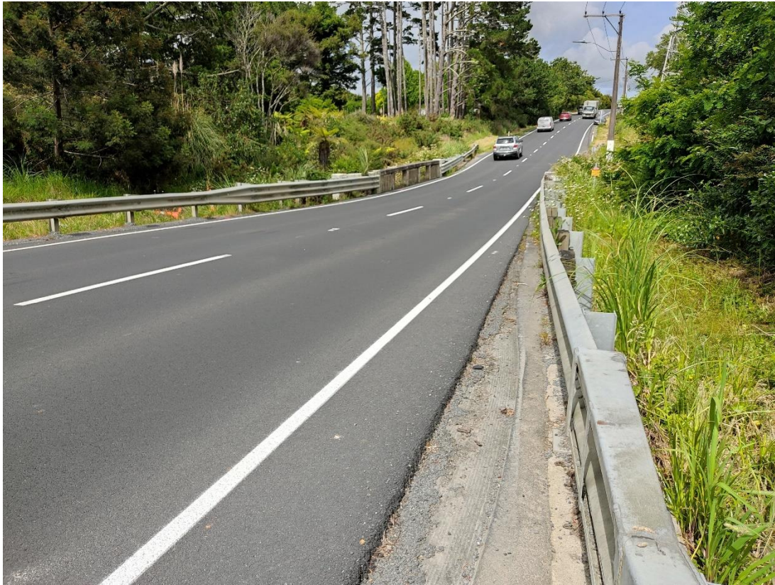
Figure 20: Narrow bridge over the Totara Creek.
