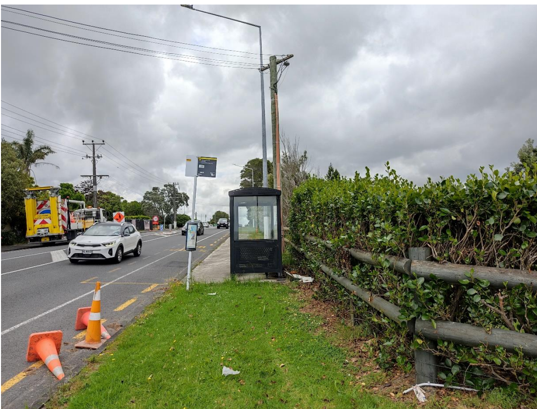
Figure 55: Current road reserve at '008'.
