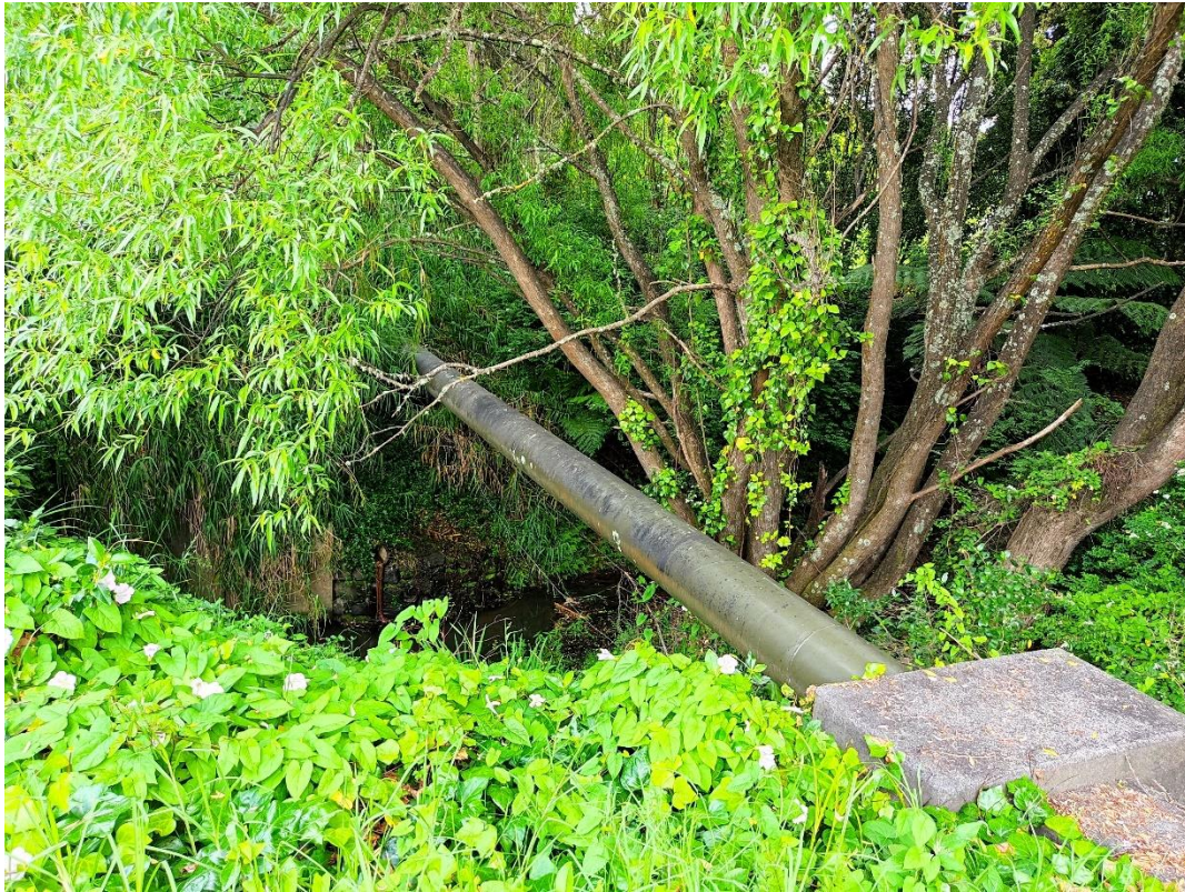
Figure 25: View over stream crossing looking downstream.
