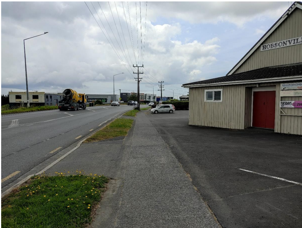
Figure 43: Hobsonville Hall in relation to the road.
