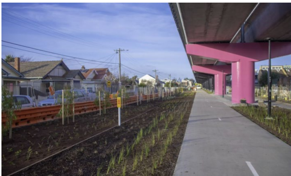
Figure 5-1: Improved cycleways under the Upfield Line.
