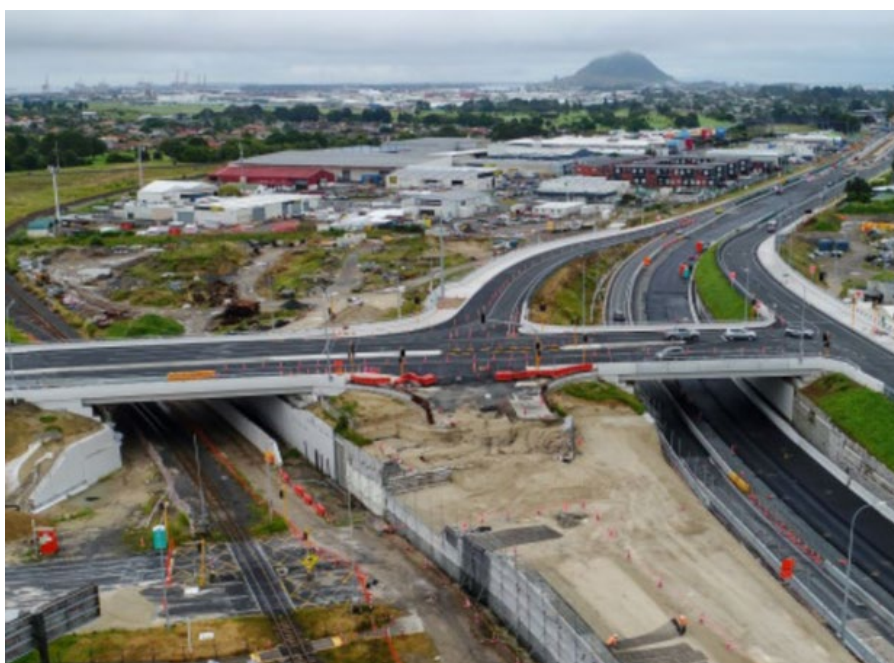
Figure 5-5: Te Maunga interchange construction
