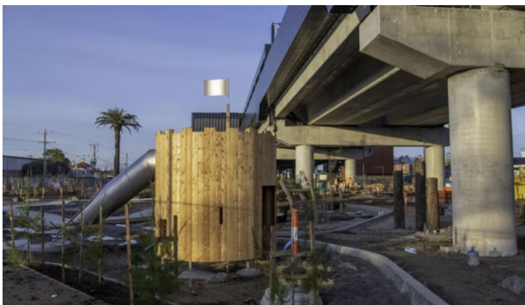
Figure 5-2: A new playground under the elevated rail line.
