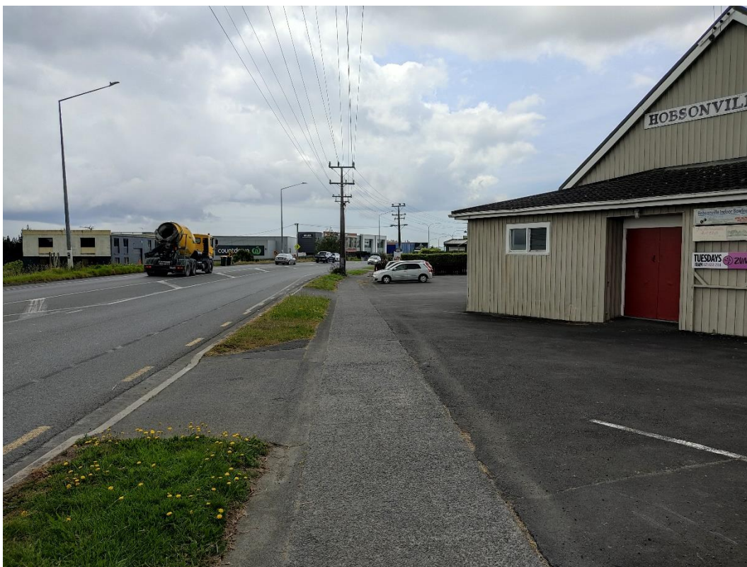
Figure 43: Hobsonville Hall in relation to the road.
