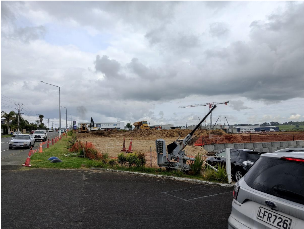
Figure 52: Recent earthworks on recorded 'gum digger camp' (003).
