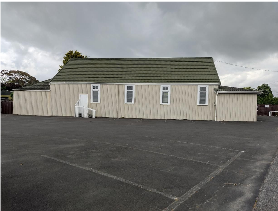
Figure 45: View over Hobsonville Hall from the carpark.
