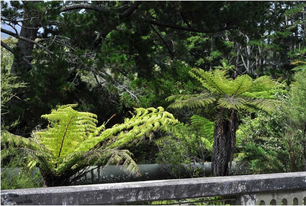
Figure 18: Totara Creek crossing, view upstream.
