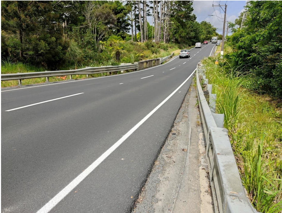
Figure 20: Narrow bridge over the Totara Creek.
