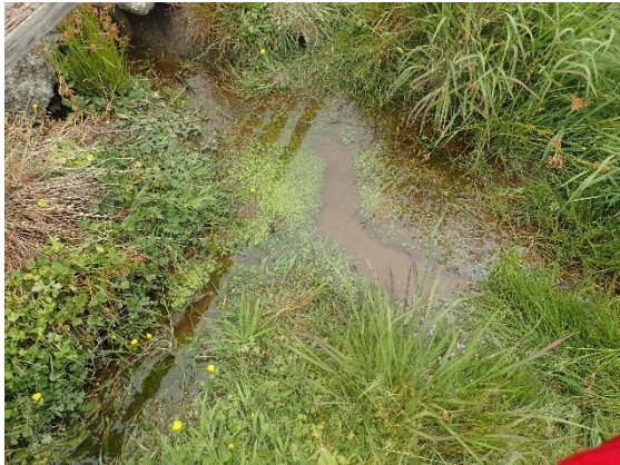
Photo 17. 9 – a pool upstream of a culvert
