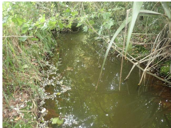
Photo 4. 2 – the stream was very deep near the culvert.
