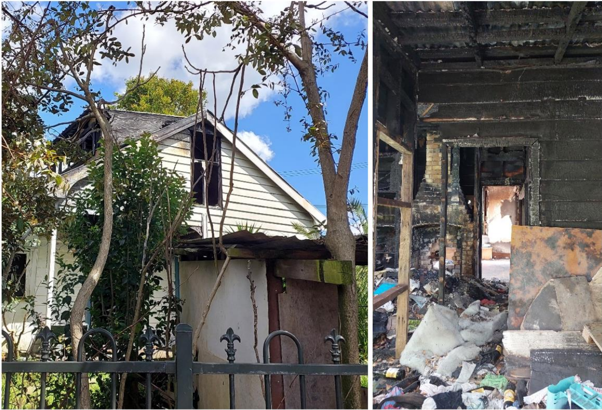
Figure 4 Unscheduled Recorded Built Heritage – Former Gardener's Cottage (CHI ref 2216) and landscaping to boundary
