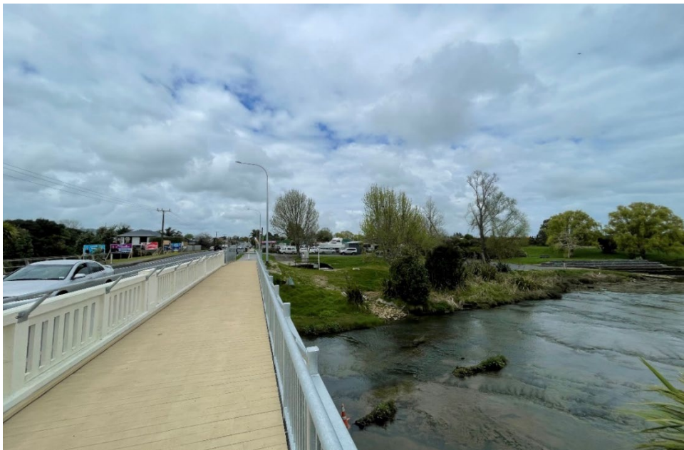
Figure 5-5: Image of the existing Otūwairoa bridge and adjacent bank to the south (Source: MJ_IGL)
