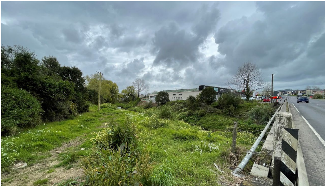
Figure 5-8: Image of the existing Hingaia bridge and adjacent bank to the north (Source: MJ_IGL)
