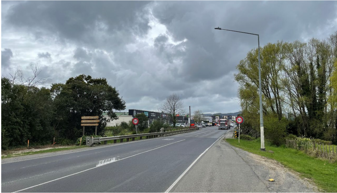
Figure 5-7: Image of the existing Hingaia bridge (Source: MJ_IGL)
