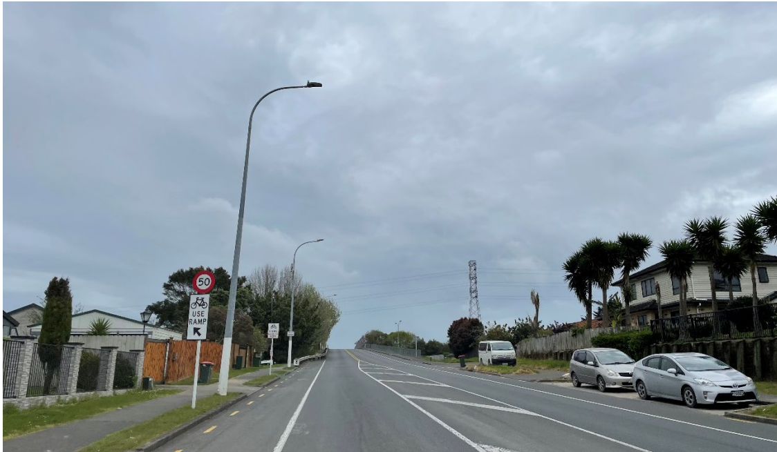
Figure 5-13: Image of the rise to the existing bridge across SH1 along Alfriston Road (Source: MJ_IGL)
