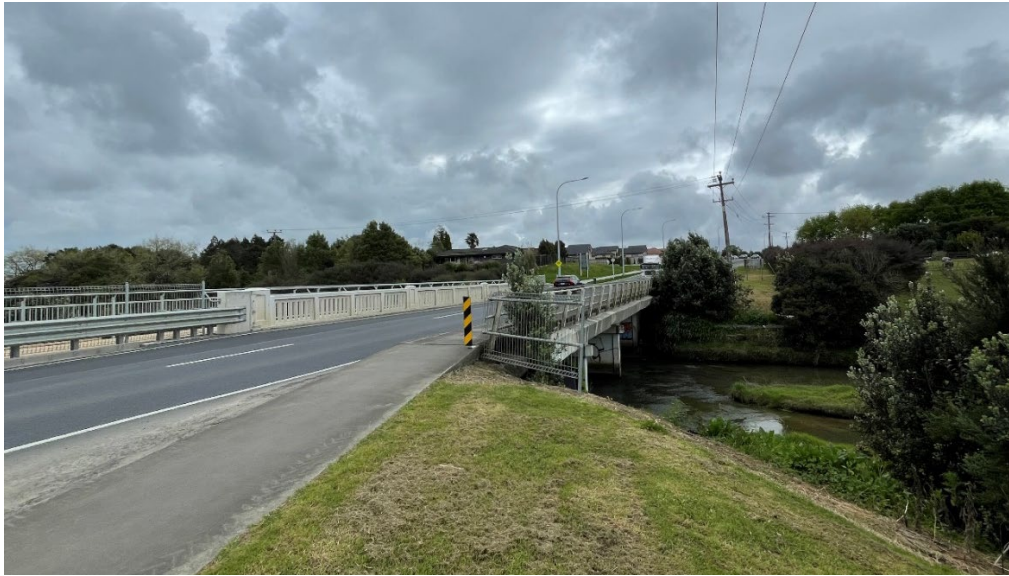
Figure 5-4: Image of the existing Otūwairoa bridge (Source: MJ_IGL)
