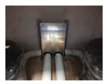
Figure 3 - Typical Outlet Weir Wall
