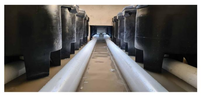
Figure 1 - AtlanFilters in a concrete chamber / vault
