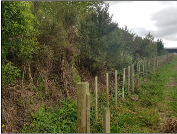
Photo 3: Planted earth bund within 787 KC Hwy.
