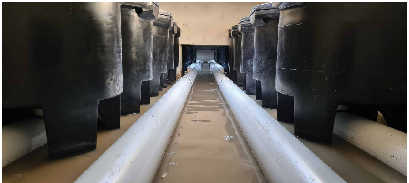
Figure 1 - AtlanFilters in a concrete chamber / vault
