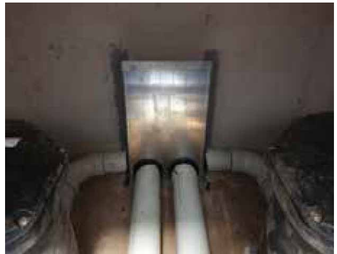
Figure 3 - Typical Outlet Weir Wall
