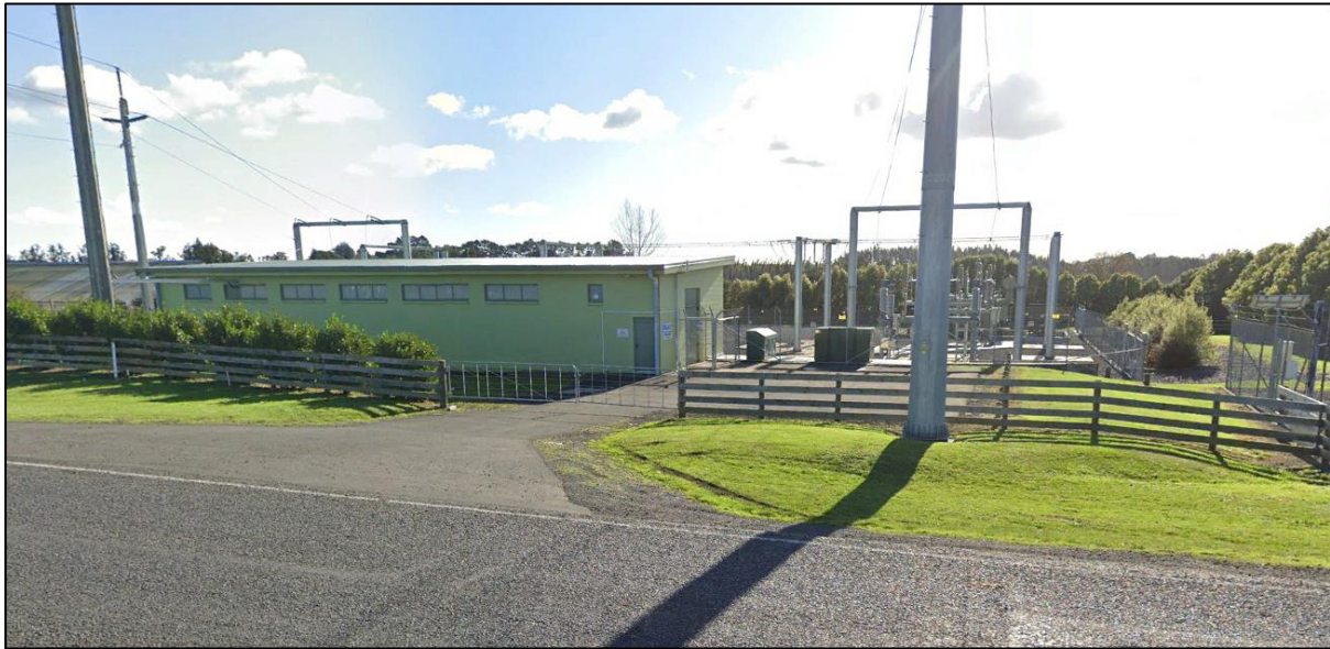
Figure 12 Example Tuakau substation, which includes a switch room, BUS structures and transformers on concrete plinths, with mitigation planting around the boundary.
