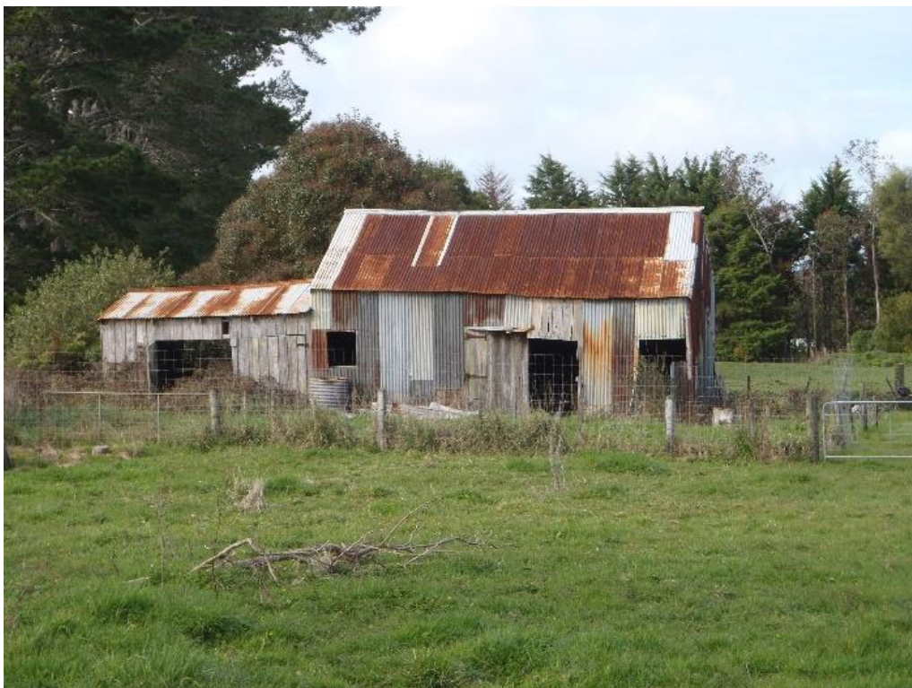
Figure 16. Corrugated iron barn at 787 Kaipara Coast Highway, now removed (from Jones and Phear 2016)
