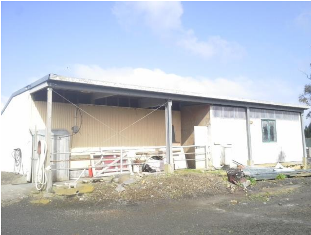
Figure 15. Farm building at 787 Kaipara Coast Highway, now removed (from Jones and Phear 2016)
