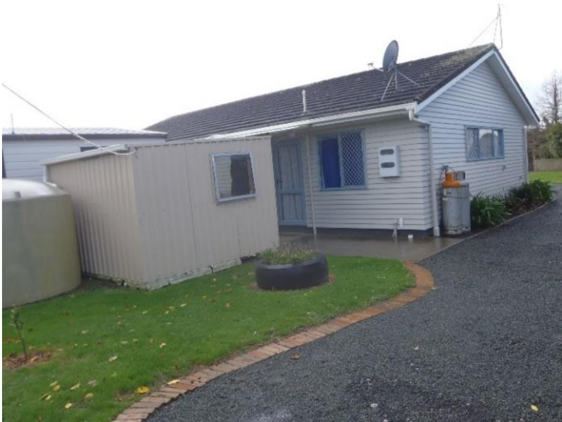
Figure 14. Second house at 787 Kaipara Coast Highway, now removed (from Jones and Phear 2016)
