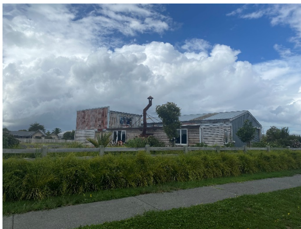
Photo 9: Eastern area of 787 Kaipara Coast Hwy
