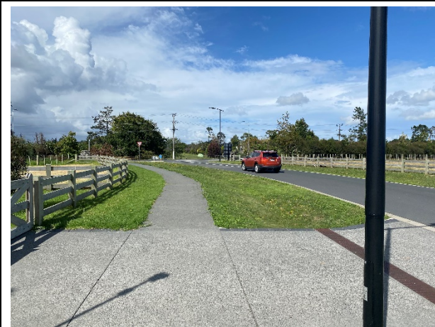
Photo 1: New access road into the Site at 787 Kaipara Coast
