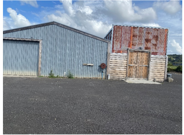
Photo 8: Site structures at 787 Kaipara Coast Hwy, eastern area.
