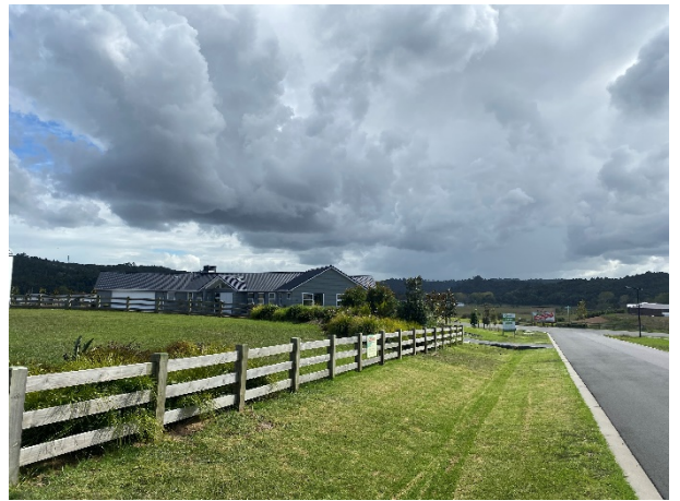
Photo 14: New landscaping and berm area at 787 Kaipara Coast Hwy.
