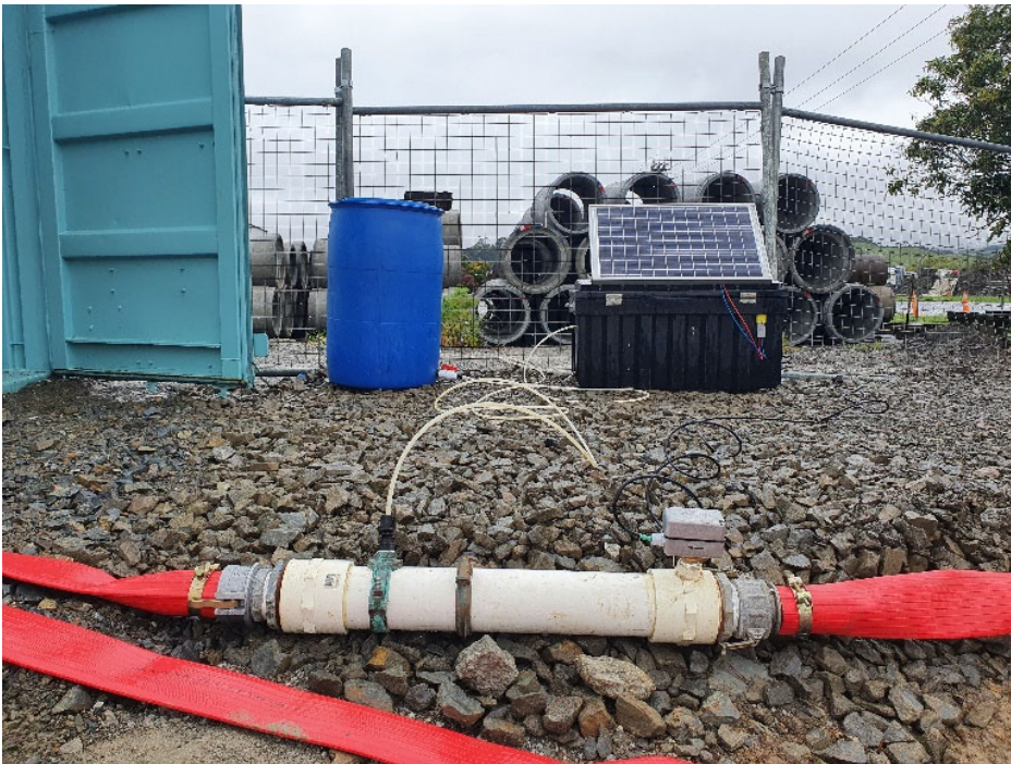
Figure 4: Example of an in-line electronic chemical dosing system (Source: Erosion Control).
