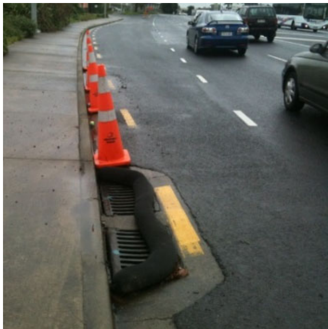
Figure 7 Example of Cesspit Protection
