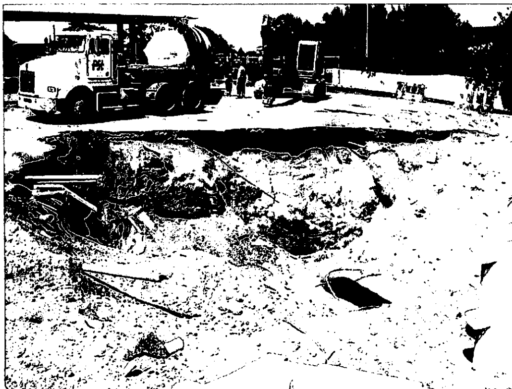
Photograph 4: The tank pit following the removal of Tank 3. The water within the base of the pit was standing water.
