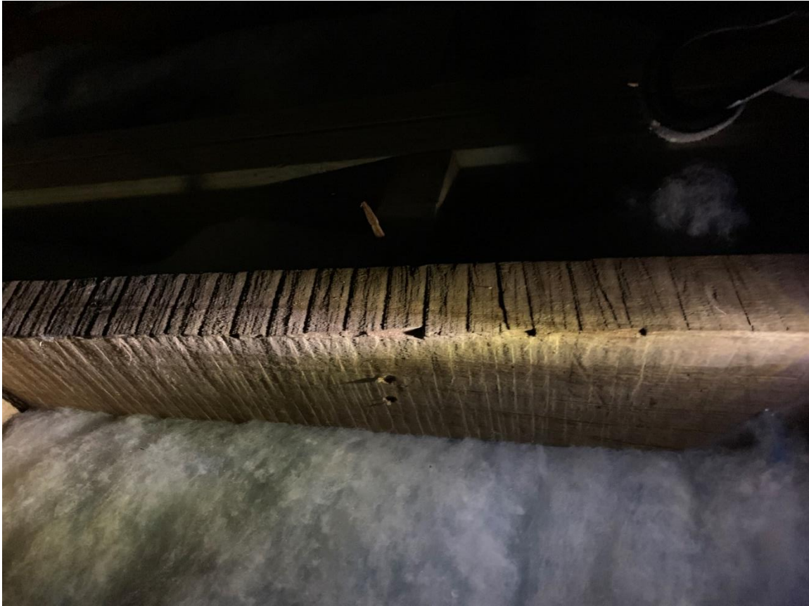
Figure 26: Pit sawn joist. Matthews & Matthews Architects Ltd, January 2019.
