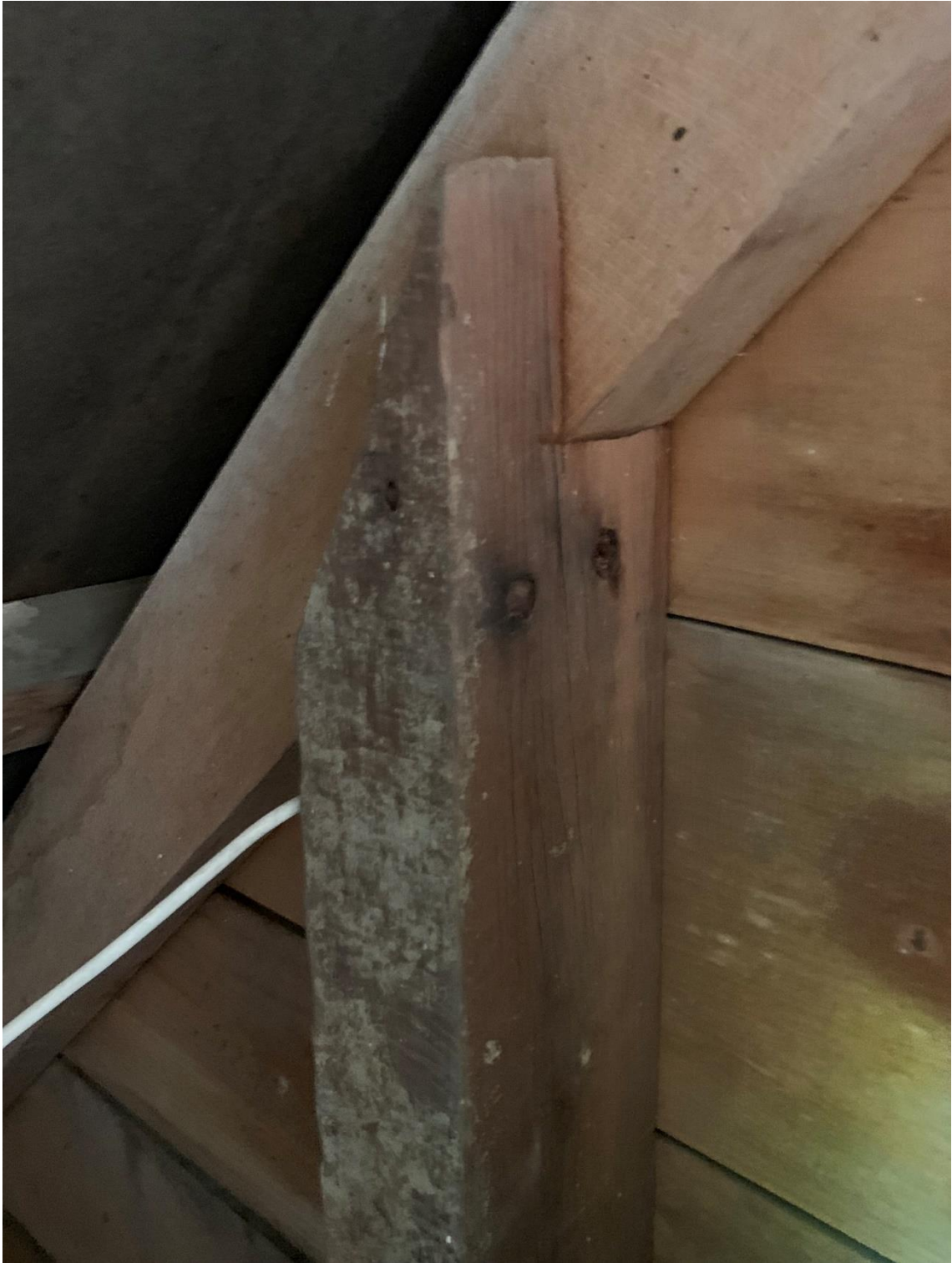
Figure 25: Pit sawn framing timber to gable end. Matthews & Matthews Architects Ltd, January 2019.
