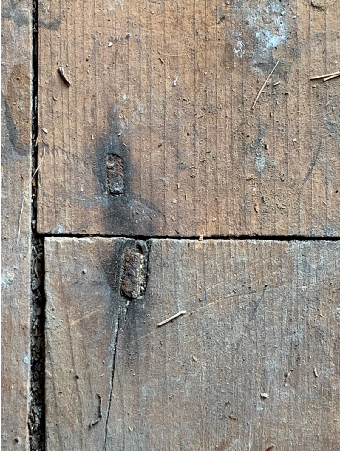
Figure 24: Early cut nails used to fix the timber floorboards in the attic. Matthews & Matthews Architects Ltd, January 2019.
