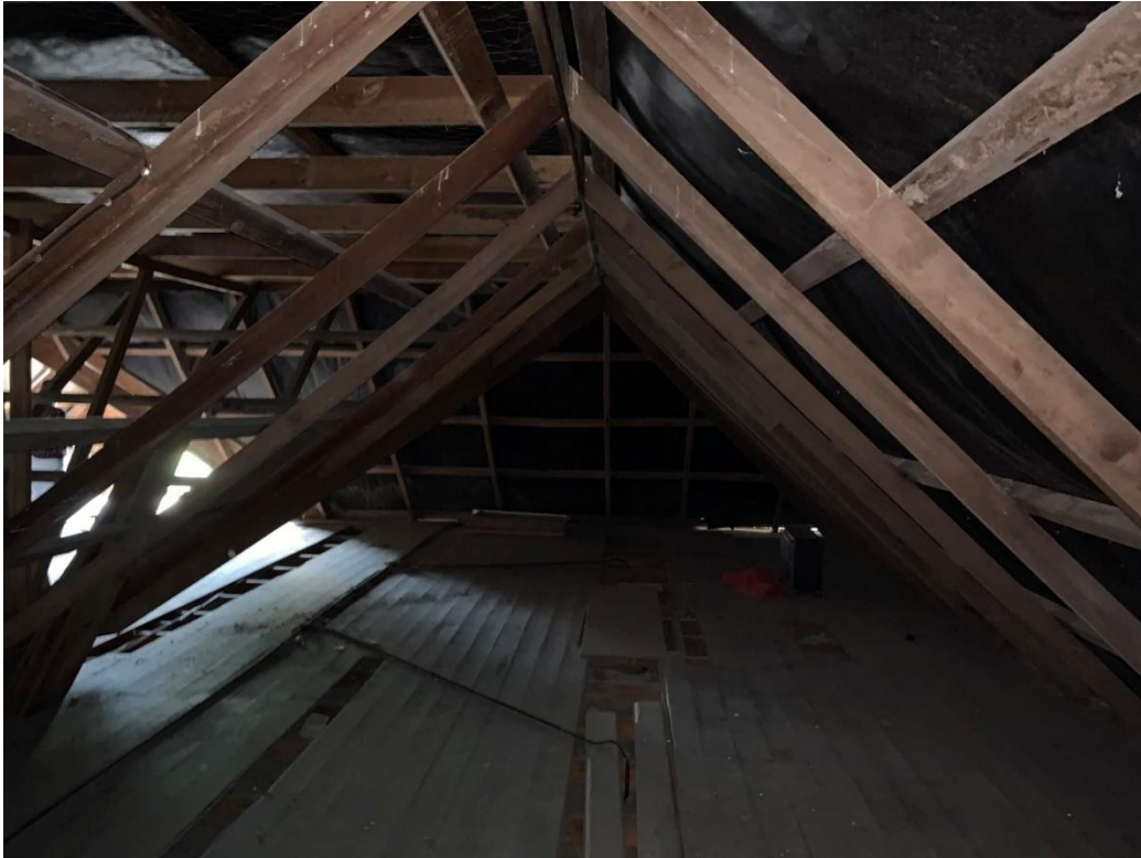
Figure 22: View north in the east side of the attic, with early timber floor boards, uplifted in some places for installation of wiring and overlaid in places with electrical conduit. Matthews & Matthews Architects Ltd, January 2019.
