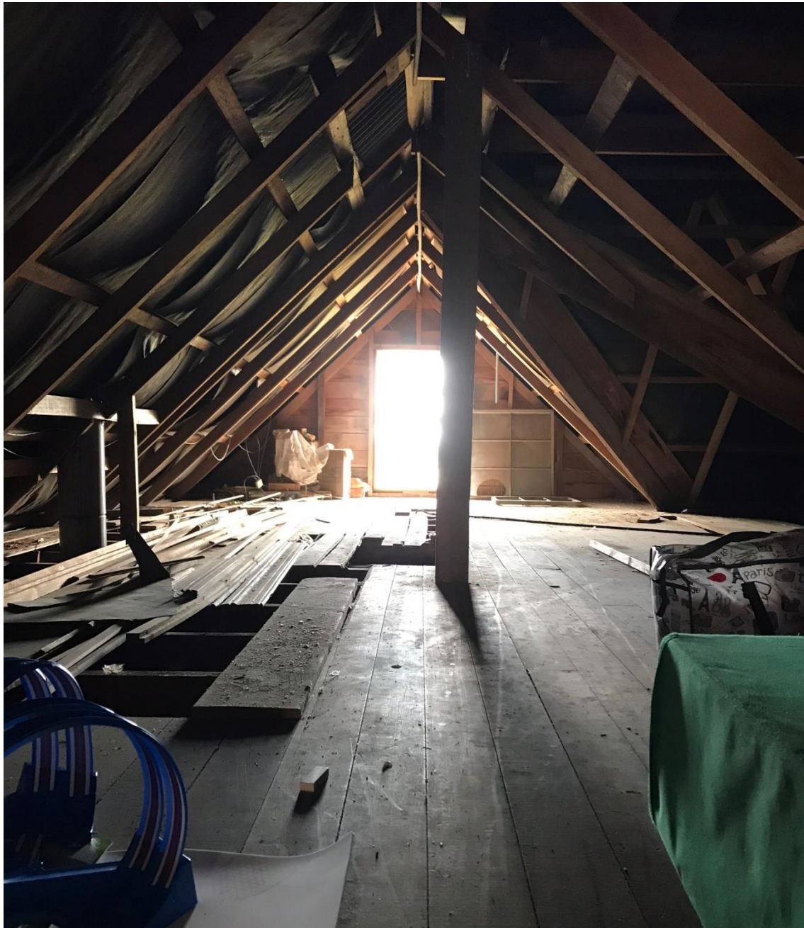
Figure 21: View north inside the west side of the attic, with early timber floor boards, uplifted in some places for installation of wiring and where chimney has been removed. Matthews & Matthews Architects Ltd, January 2019.
