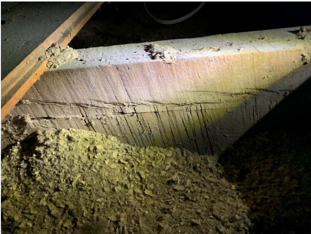
Figure 23: Pit sawn joist and early saw dust insulation. Matthews & Matthews Architects Ltd, January 2019.
