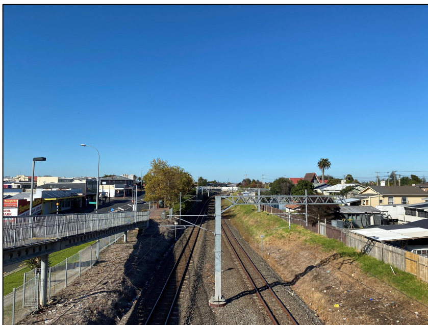
Figure 4-8: NIMT looking south from Papatoetoe Station
