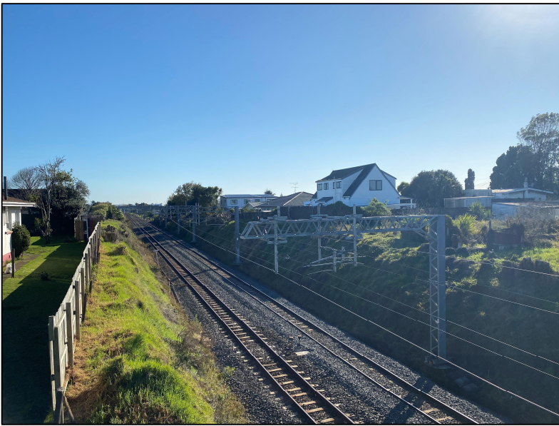
Figure 4-10: View North from Bridge Street
