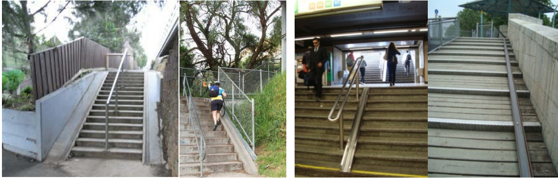
Figure 81: Examples of cycle wheeling ramps (sources: Bike Victoria and AT) 2 pictures onleft - concrete wheeling ramps as integral part of stairways, 2 pictures on right - retrofitted cycle wheeling ramp options
