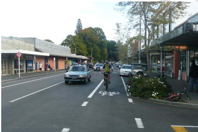
Figure 44: Cycle lane next to parallel parking
