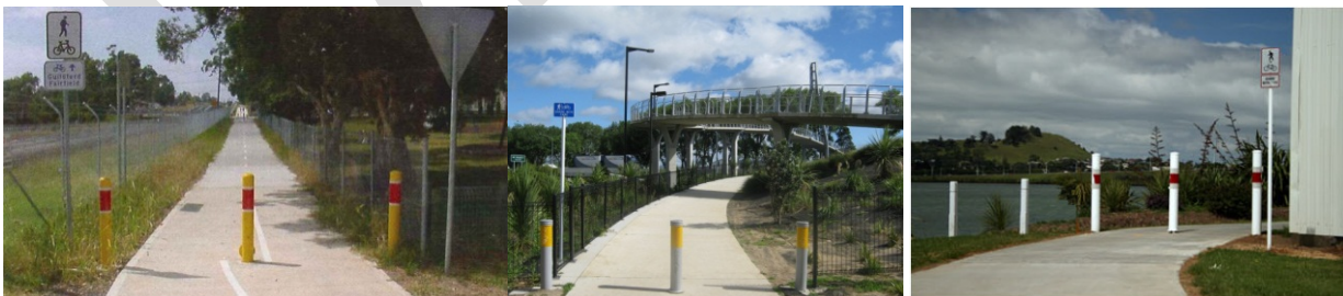
Figure 76: Examples of bollards on shared path from left to right: Austroads (2009m) SH 20 cycleway near Ketih Hay Park (Akl), Waikaraka cycleway (Akl)
