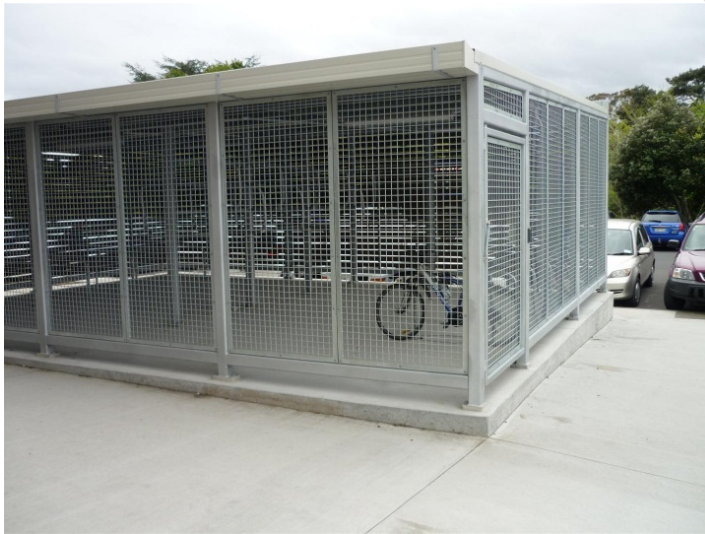
Figure 99: Cycle Parking Cage - Middlemore Hospital (K Hancock)
