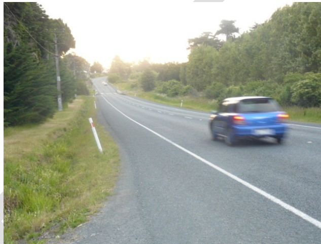
Figure 58: Sealed shoulder, SH16, Akl
