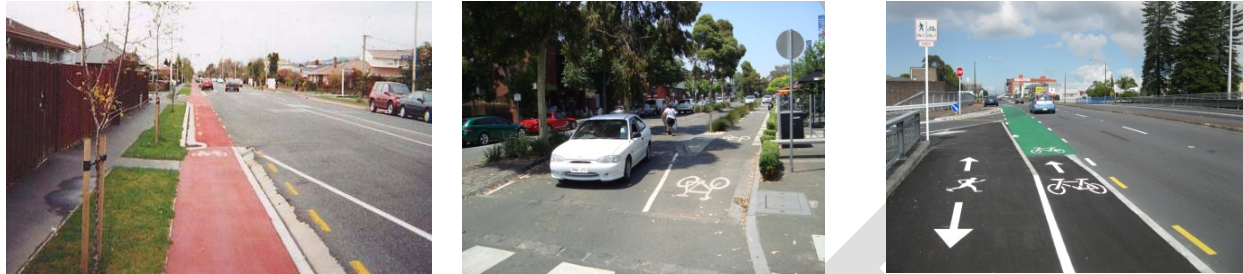
Figure 63: Examples of cycle path converting to cycle lane to give cyclists priority through intersection (from left to right; Christchurch, Melbourne, Auckland Ian McKinnon Drive)
