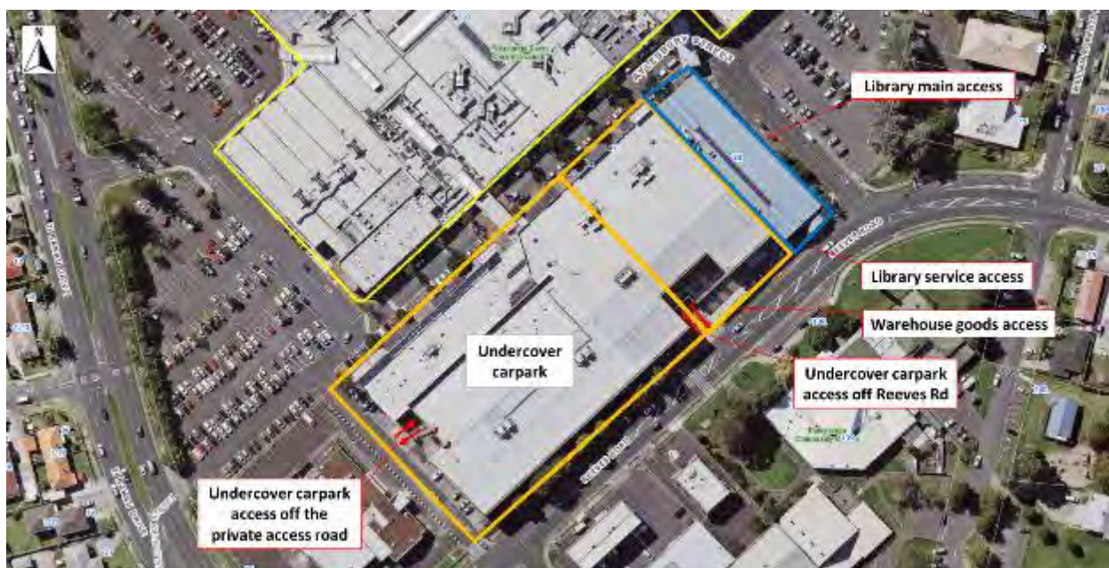
Figure 78: Pakuranga Plaza undercover carpark accesses
