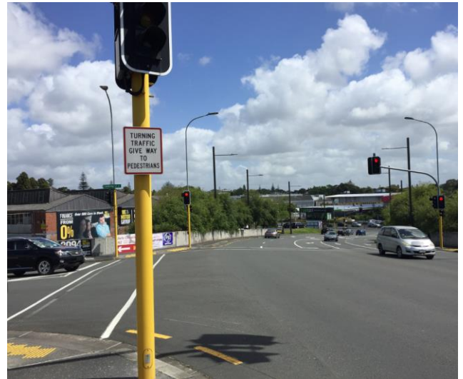
Figure 2-5 Clark Street and Cambridge Lane intersection (looking towards Great North Road) (photo taken at 11:30 am on 31-10-2019)
