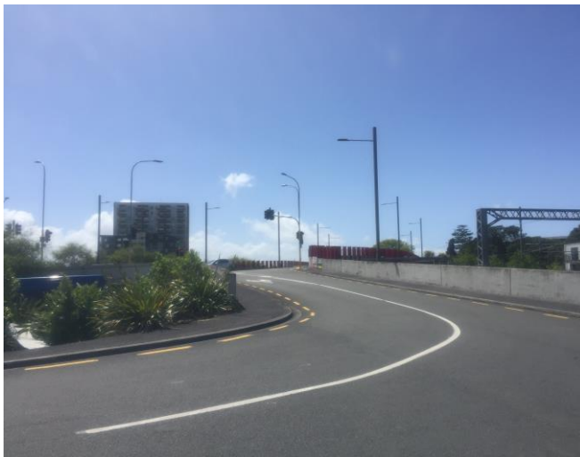
Figure 2-6 Cambridge Lane (looking east towards the Clark Street intersection and overbridge) (photo taken at 11:30 am on 31-10-2019)
