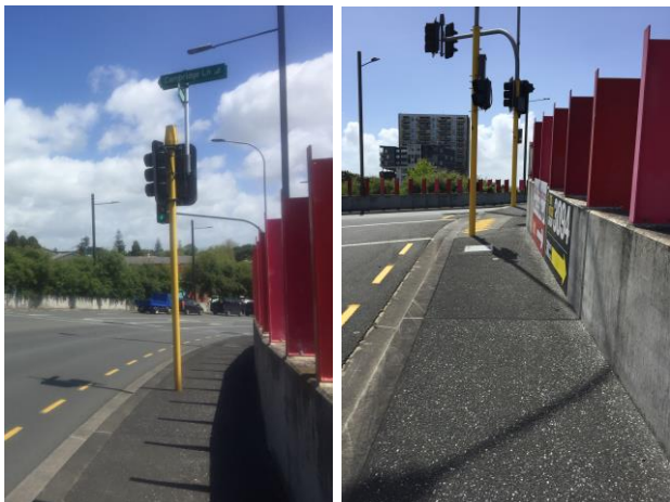
Figure 5-2 Localised narrowing of Cambridge Lane and Clark Street footpaths at the intersection to the site access (photo taken at 11:30 am on 31-10-2019)
