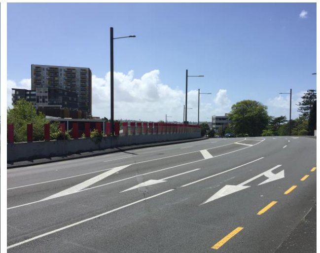
Figure 2-7 Clark Street overbridge (photo taken at 11:30 am on 31-10-2019)
