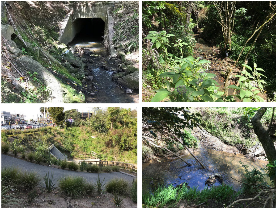
Figure 4: Manawa Stream (Clockwise from top left: Outlet of the Manawa Stream culvert beneath Railway line; typical stream reach through the site; confluence of Manawa and Scroggy streams; Inlet of the Manawa Stream culvert beneath Great North Road)
