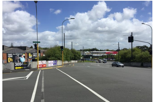
Figure 2-10 Cambridge Lane / Clark Street intersection pedestrian crossing (looking toward Great North Road) (photo taken at 11:30 am on 31-10-2019)
