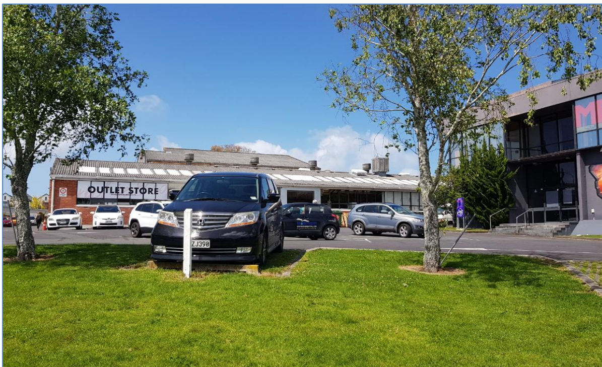
Figure 2: Photo of Existing Buildings
