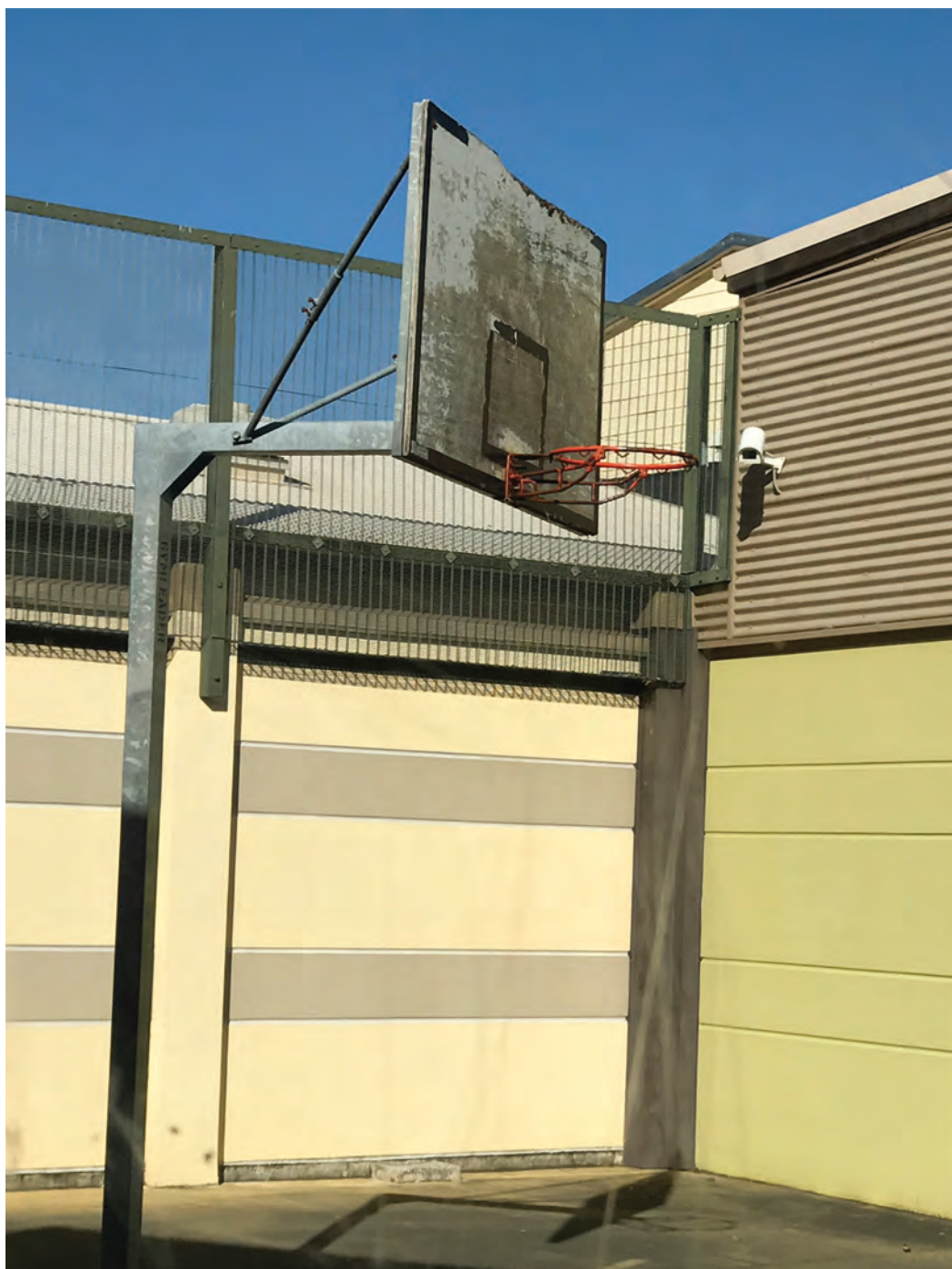
Photo 10 Basketball court at a care and protection residence
