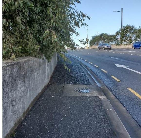
Figure 3-4 Overhanging planting from adjacent property reduces effective footpath width on the northern side of Clark Street
