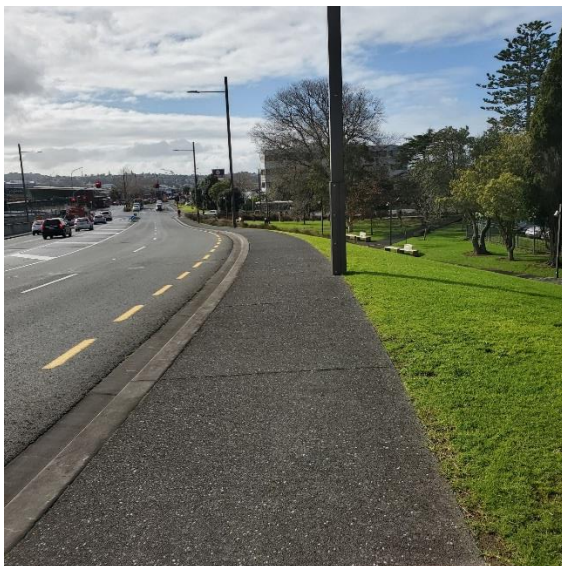
Figure 3-5 Southern footpath on Clark Street toward Rankin Avenue
