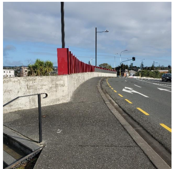
Figure 3-6 Critical section of the footpath on the southern side of Clark Street
