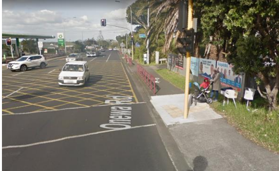
Figure 3-9 Pedestrian railings installed on Onewa Road alongside a narrow shared path in close proximity to Northcote Primary School
