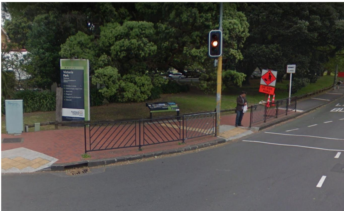
Figure 3-11 Safety barriers used to guide pedestrians to formalised crossing points on Fanshawe Street and provide separation between the footpath and adjacent traffic lane
