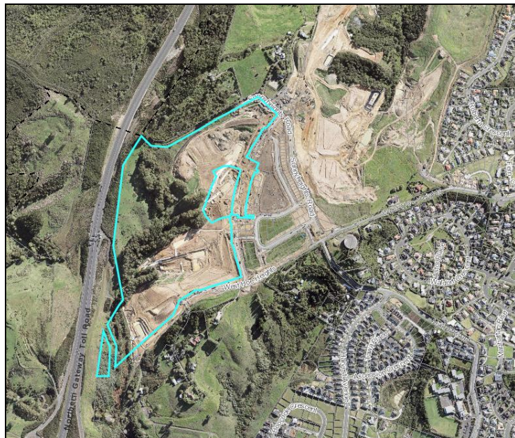
Figure 1 – Greater Site Aerial
