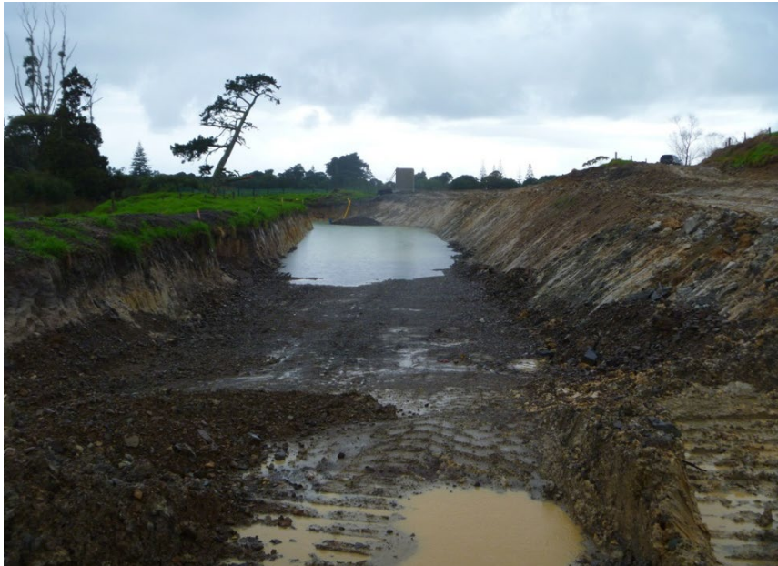
Figure 12 – Shear Key excavation
