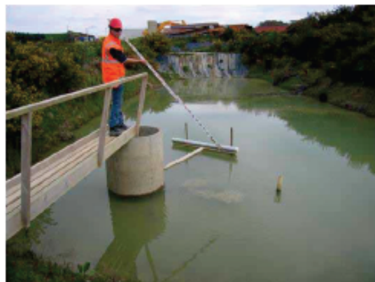
Undertaking Maintenance of a Sediment Retention Pond
