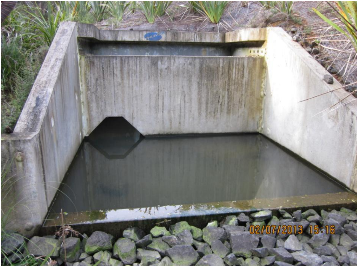
Photo 1 – Impact basin on NGTR Otanerua Wetland outfall
