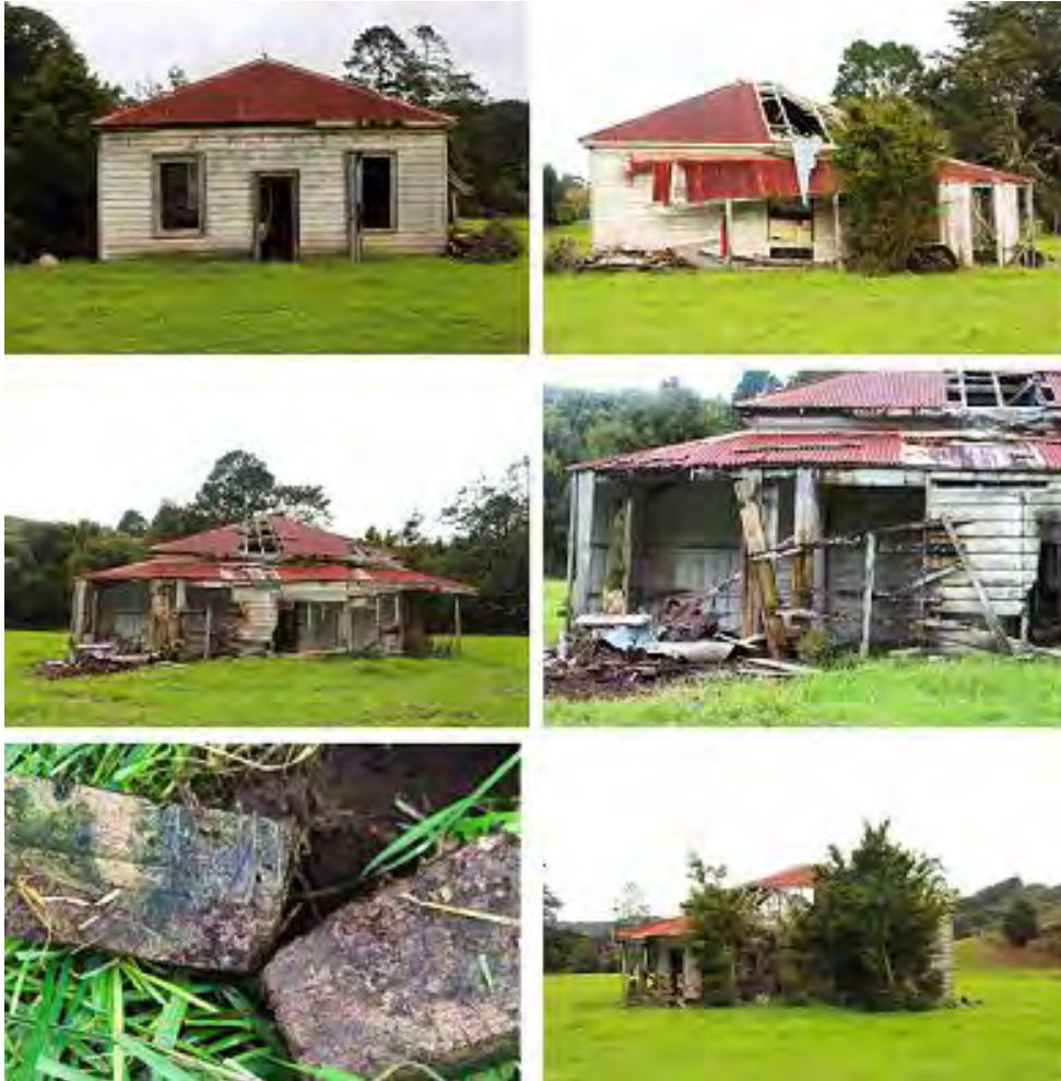
Figure 80 – Woodthorpe exterior. Top (left) looking W front elevation and (right) looking S at verandah on north elevation; Middle (left) looking E at lean-to and (right) looking E at N end of lean-to ; Bottom (left) wire cut bricks from the original chimney now gone and (right) looking N at southern elevation
