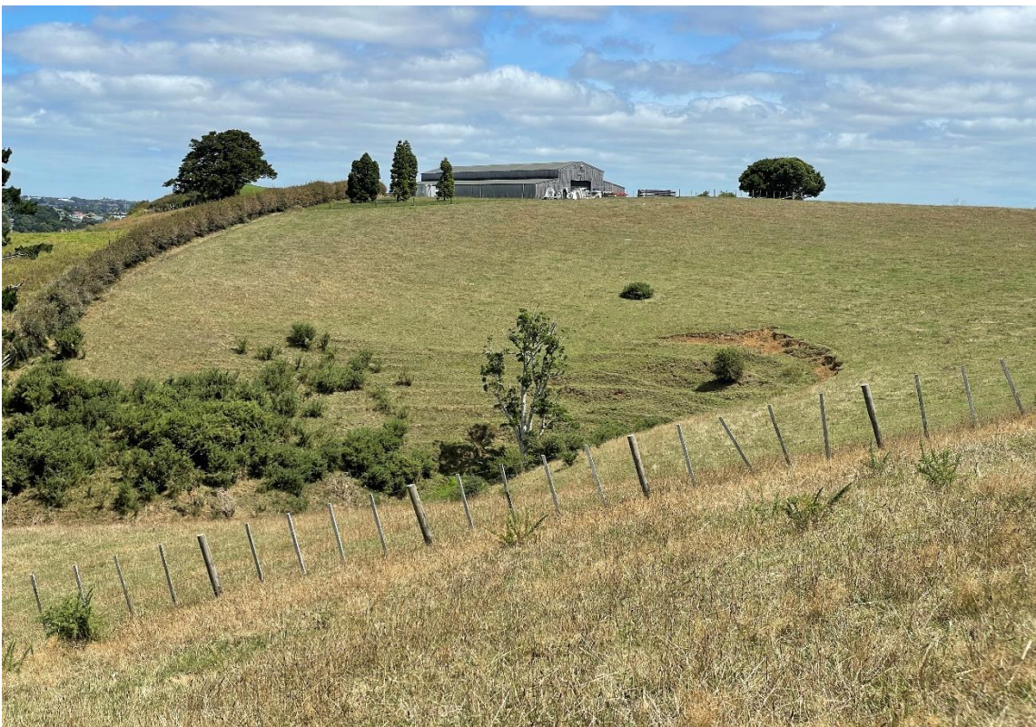
Photo 4: Typical steep slope with arcuate slip beneath ridgeline.
