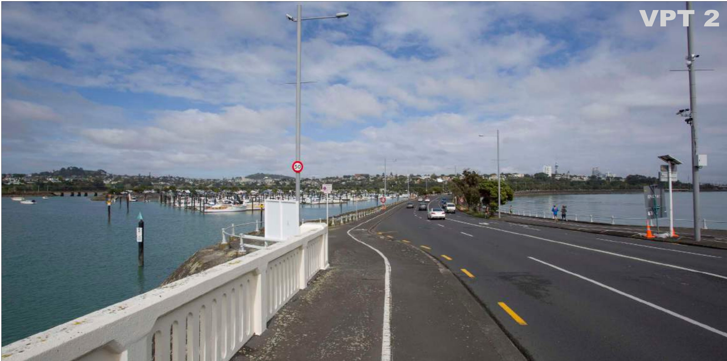
GEORGE STREET APARTMENTS. PHOTOGRAPH VPT 2 VIEWED FROM TAMAKI DRIVE
