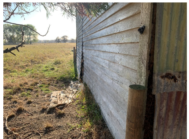
Photo 12: Northern exterior of the shed pictured in Photo 9.
