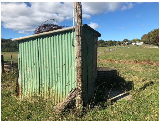
Photo 21: Pump shed in south-western portion of the site adjacent to current accessway.
