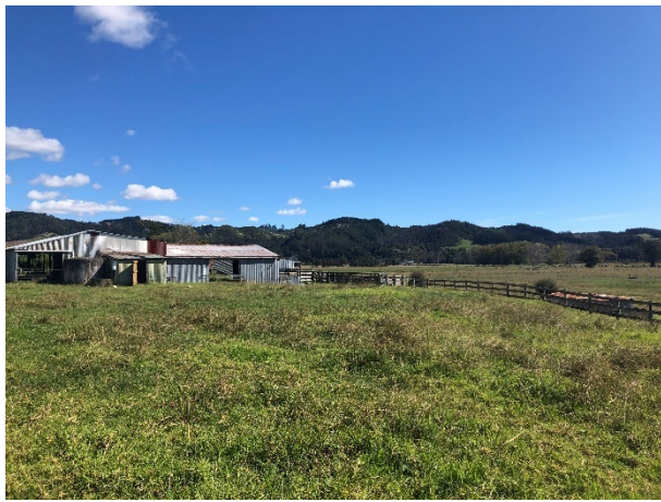
Photo 27: Building associated with stock yards in south-eastern portion of the site. Photo taken facing south west.
