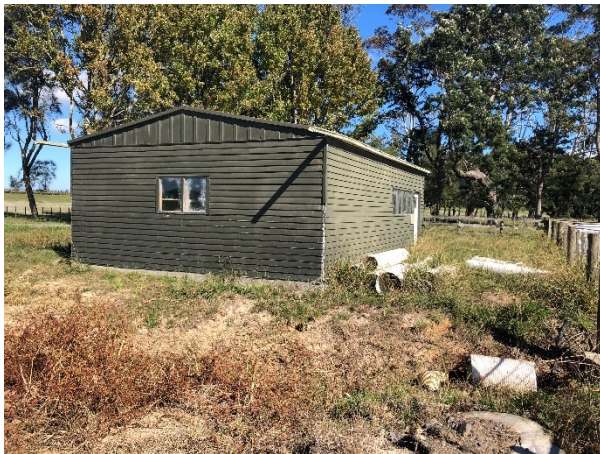
Photo 33: Green steel shed/disused pipes in the western portion of the site, south east of the large white barn. Photo taken facing west.
