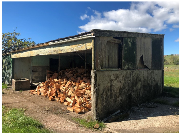
Photo 14: Shed in south western portion of site adjacent to current accessway. Cladding of building is constructed of potential ACM. Photo taken facing south east.
