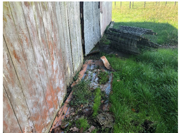
Photo 20: Disused corrugated iron, timber and wire adjacent to southern side of building constructed of potential ACM, as pictured in Photo 12.
