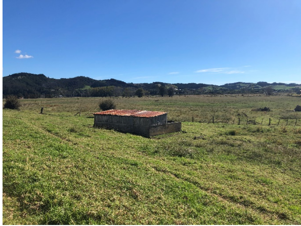
Photo 31: Concrete building with corrugated iron roofing located within the paddock directly north of the stock yards in the south-eastern corner of the site. Photo taken facing north west.
