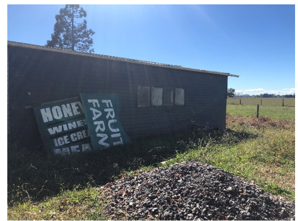
Photo 34: Southern side of building pictured in Photo 27, adjacent to a small pile of stone aggregate. Photo taken facing north west.
