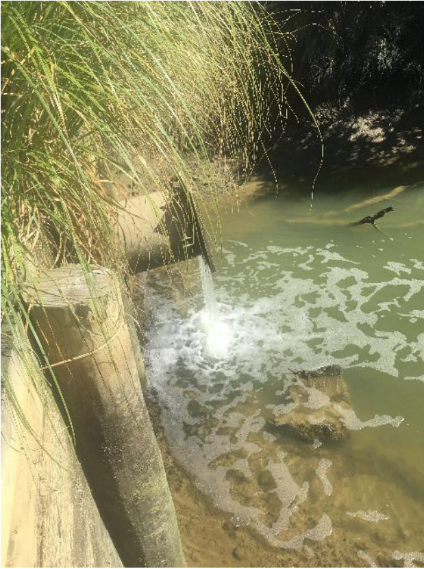
Photo 5 Culvert A (outside of development site)
