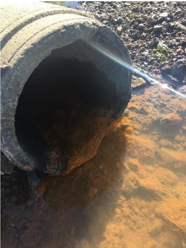
Photo 6 Culvert B (outside of development site)
