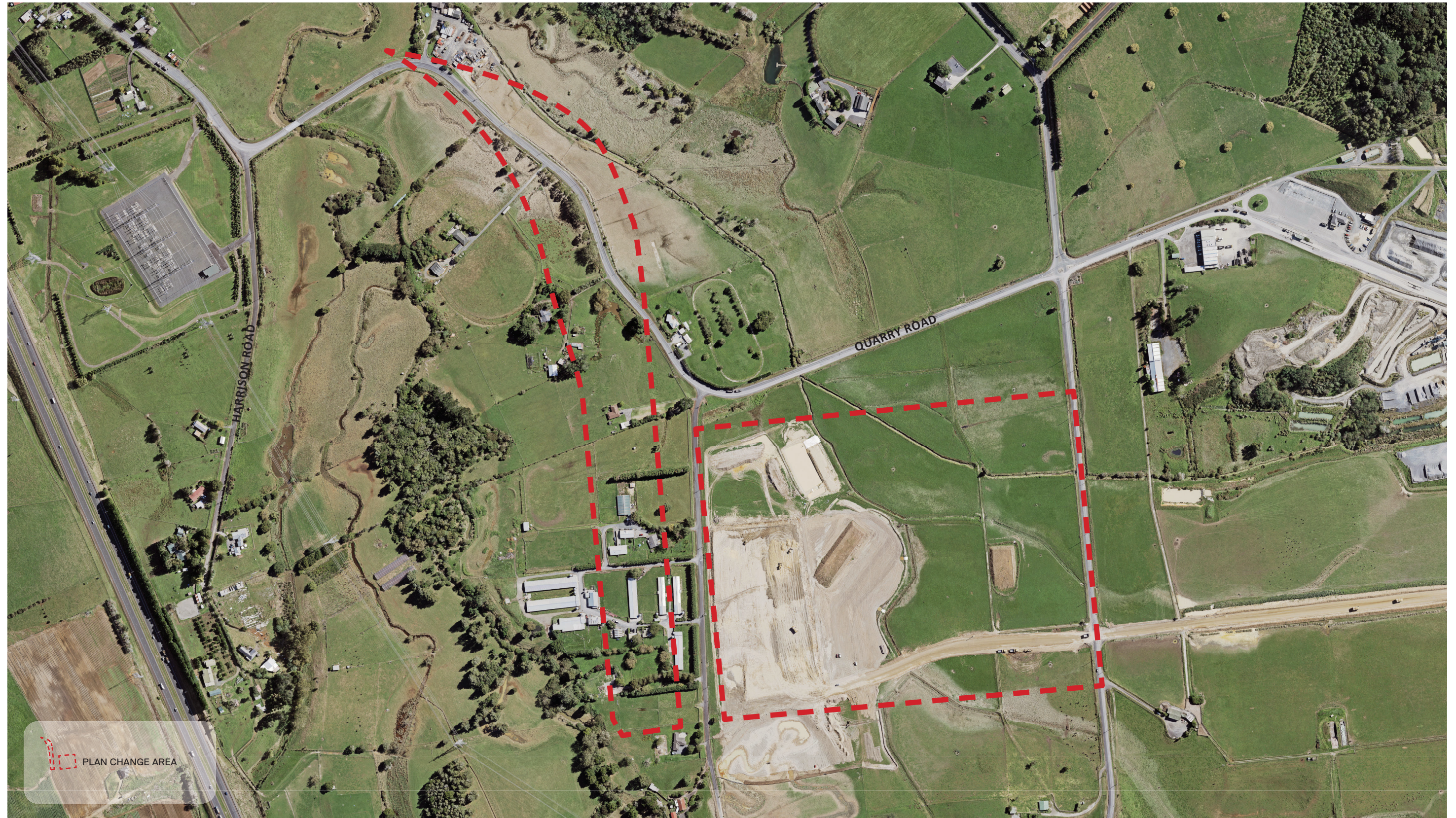
[PHOTO TAKEN BEFORE RECENT SITE EARTHWORKING]
