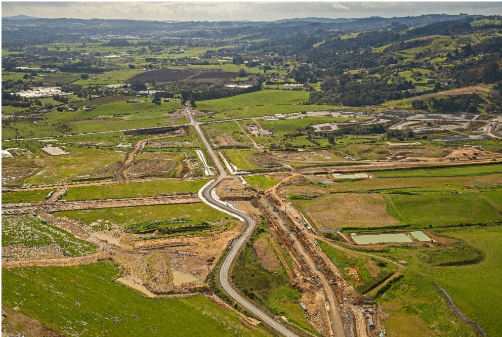
Figure 2: Showing the Drury South development as viewed from the south.
