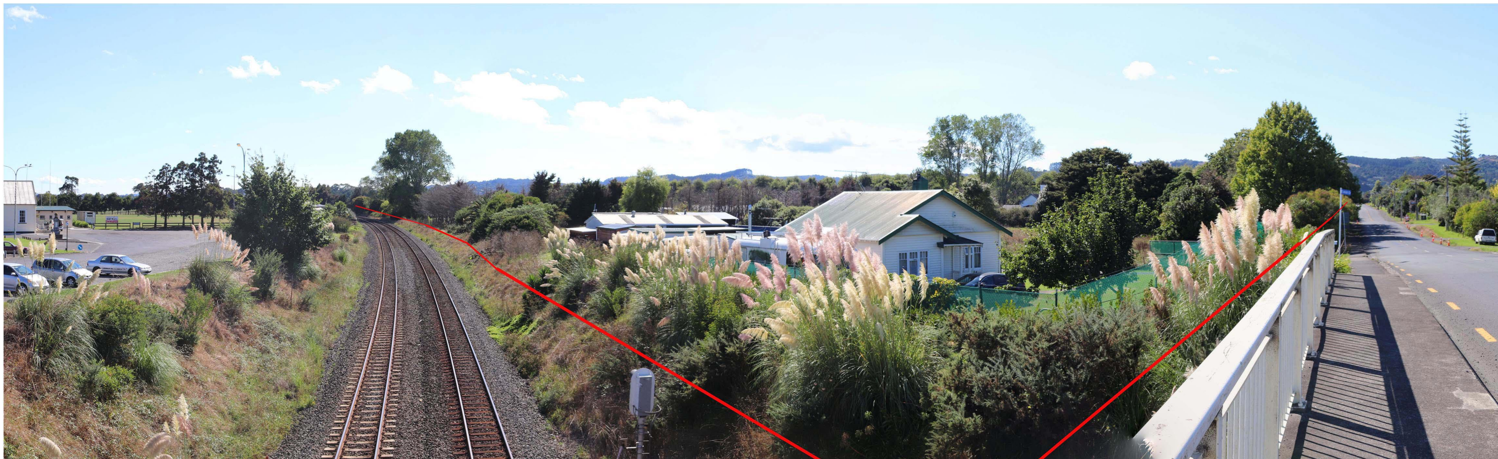
Photo-Viewpoint 3 (from the Waihoehoe Road Rail bridge looking to the northeast)
