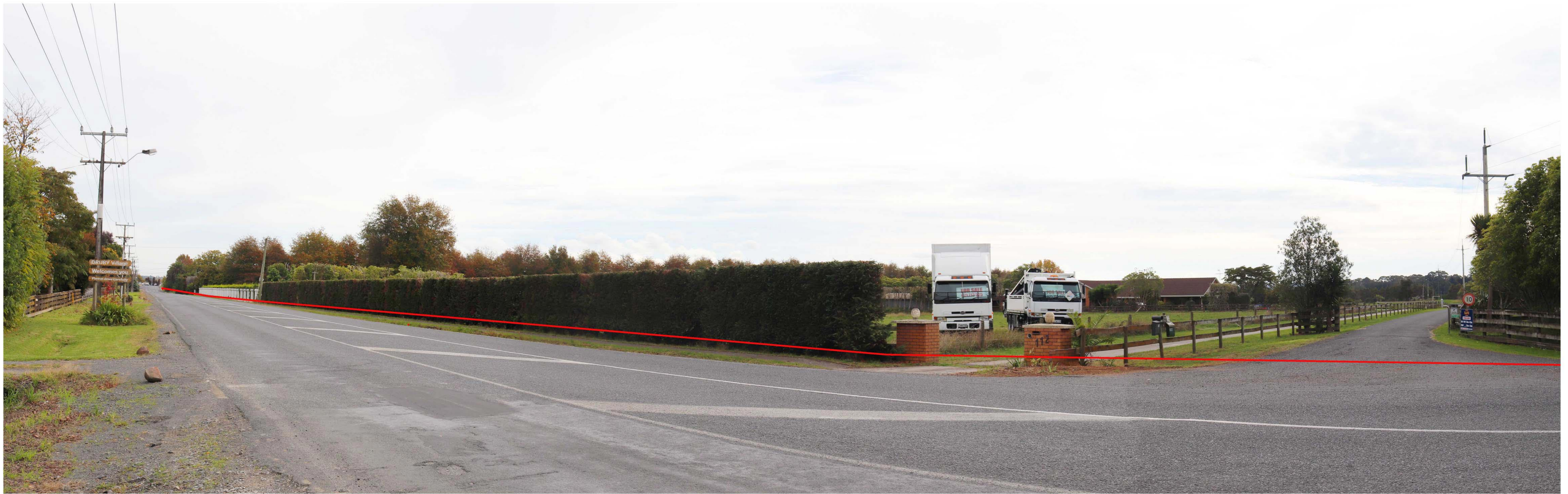
Photo-Viewpoint 1 (from near the corner of Waihoehoe Road and Fitzgerald Road looking to the northwest)
