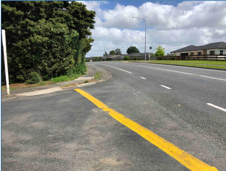
Figure 6 Great South Road looking to the south from the Gatland Road intersection
