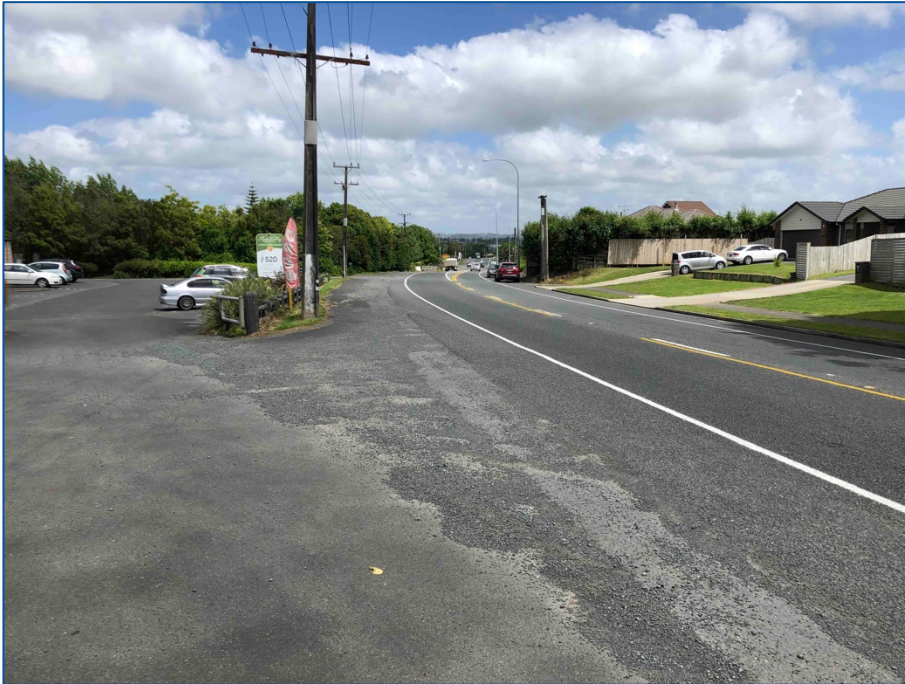
Figure 4 Great South Road looking to the south from proposed new intersection
