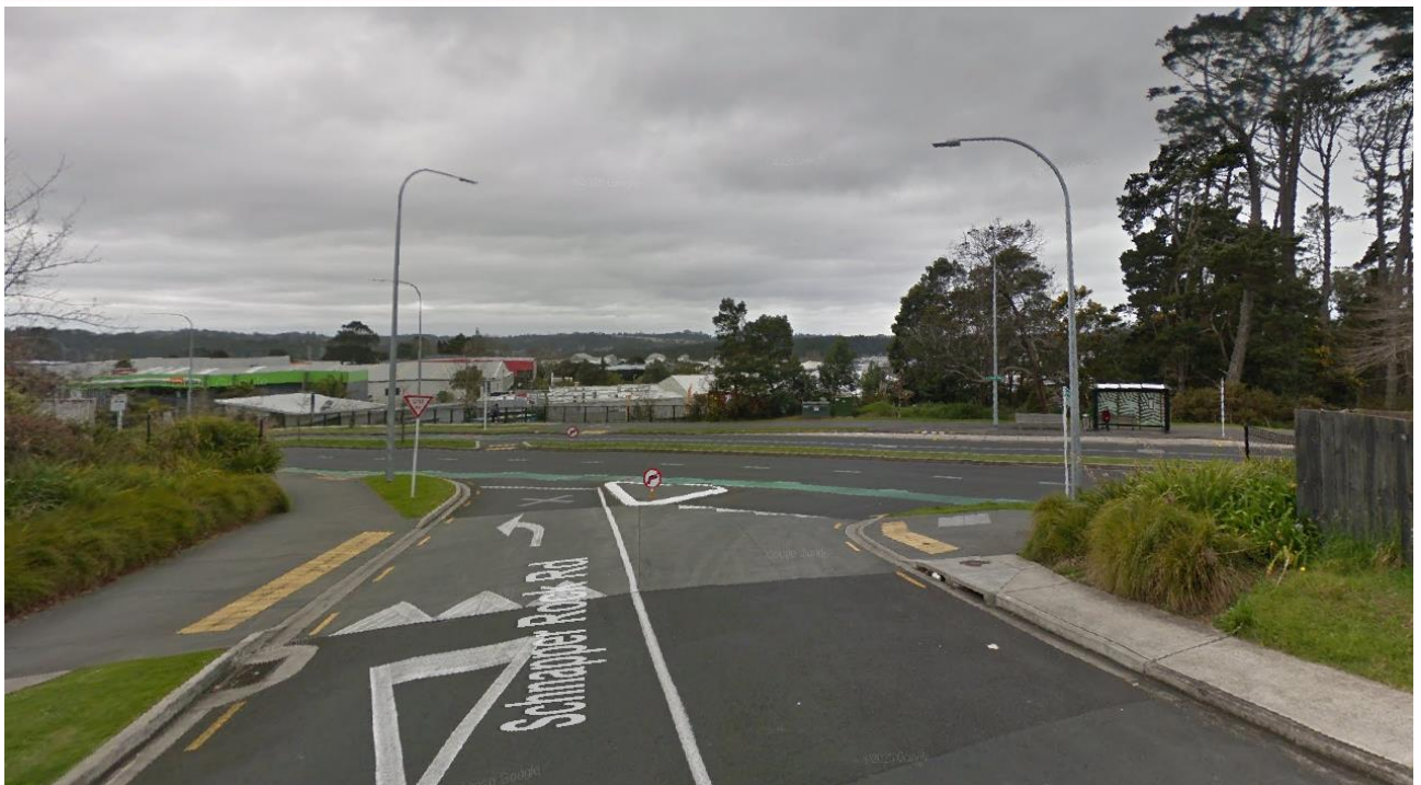
Figure 3.4 Intersection of Schnapper Rock Road and Albany Highway (north)
