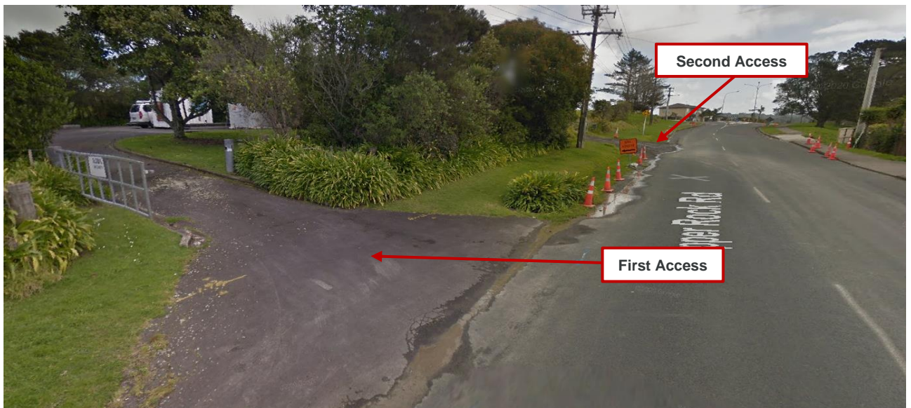
Figure 2.4 Existing site accesses
