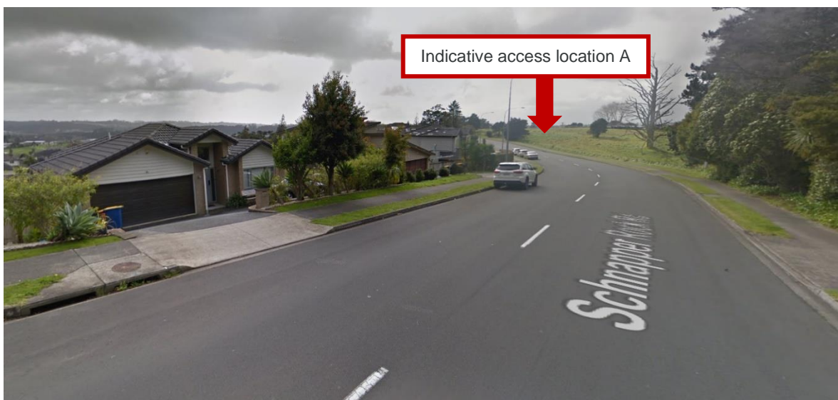
Figure 5.6 Eastbound view toward indicative intersection location (Streetview)
